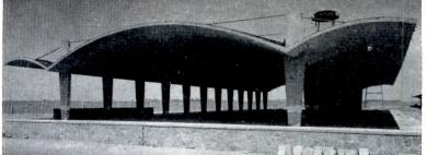
SHORT CYLINDRICAL SHELL: Mexico City Customs Warehouse. Short shells, span 66 ft; 20 ft cantilever wing; ties above roof. With Carlos Recamier, Architect.
