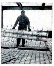
PLACING units is an easy 10-second job! E/R Cofar span ranges up to 16' and 1-, 2-or 3-cell E/R units anticipate any future electrical needs. T-wires welded to corrugations provide temperature reinforcing, mechanical anchorage between concrete and steel.
