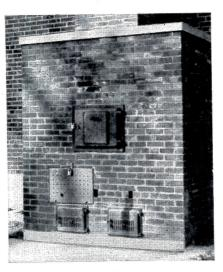
COMMERCIAL AND IN-DUSTRIAL direct-fed incinerators for on-the-spot disposal of excelsior, rubbish, etc.
