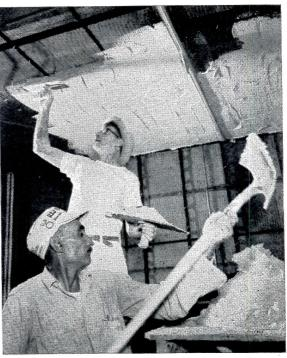
TRUSCON METAL LATH and plaster provide flexibility in ceilings that are sometimes level, sometimes domed, sometimes formed into unusual contours. And you get additional structural advantages, such as rigidity, resistance to cracking and impact, sanitation, relative lightness of weight, and long-term economy. Write today.
