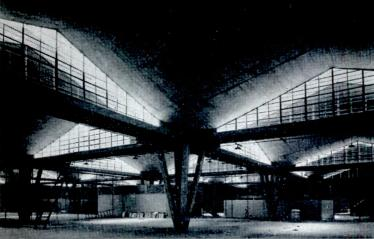
YPERBOLIC PARABOLOID (Vertical axes): Herdez Factory, Mexico, .F. Rectangular domes formed by 4 h. ps. Catwalk carries lighting and coneals ties. Span 52 by 52 ft. Vertical axis; limited by straight generators
