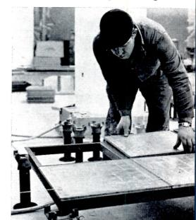
Aluminum Floating Floor plates are set in module frame, covered with standard flooring
