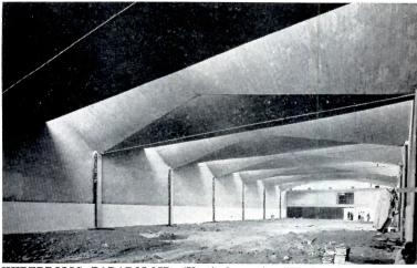
HYPERBOLIC PARABOLOID (Vertical axes): "El Leon" Confectionery Factory, Mexico, D.F. "Half-umbrellas" spanning 66 ft in sawtooth. Ties are necessary to take lateral thrusts
