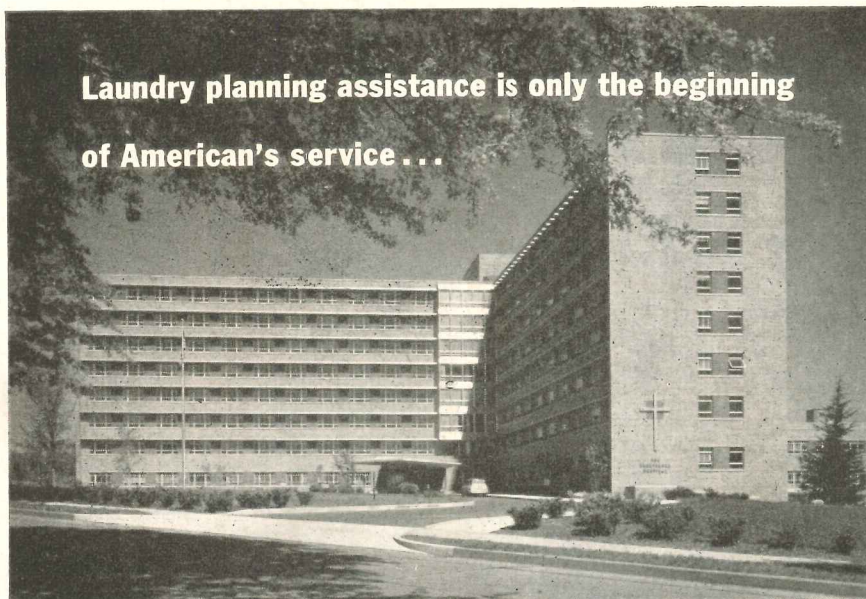
Providence Hospital, Washington, D. C. Architect: Faulkner, Kingsbury & Stenhouse. General Contractor: Charles H. Tompkins Company. Laundry Equipment: The American Laundry Machinery Company.
