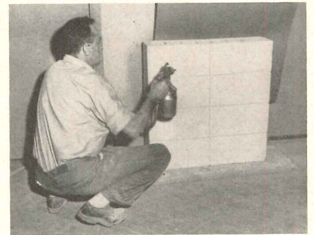
When sprayed on concrete block, thin Mozel coating retains rough texture of base
