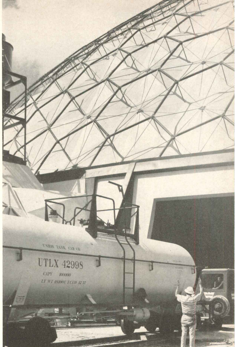
In the illustrations may be seen the usual stages involved in the handling of a tank car, from its arrival on a track outside the building, placement of the car on the rotating transfer table, and finally the transfer of the car to one of the maintenance areas
