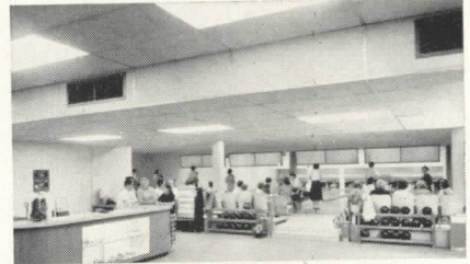
Lebanon Lanes, a part of the L.M.S. Office Building, Pittsburgh, Pa. This new building uses both Tectum roof deck and 1" suspended acoustical board. Acoustics are ideal. Designers & Builders: Larson Construction Company, Pittsburgh.
