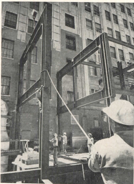
Second of two Vierendeel trusses goes into position against original building
