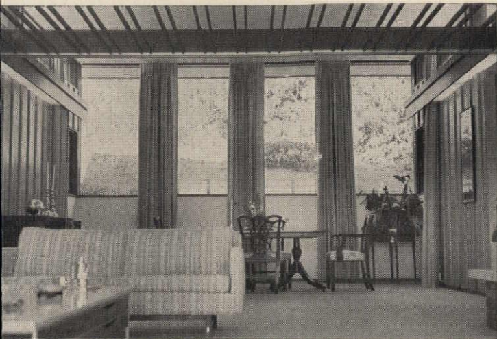
VOLK RESIDENCE, Smoke Rise, N. J. All exterior window walls were constructed of shop-built, prefabricated modular frames, all dimensioned around standard Thermopane sizes. These same panel types, which were fitted into the modular wood framing system, together forming the structural wall and exterior and interior finish, accommodate standard steel sash, blank opaque walls, French doors and regularly hinged doors.
