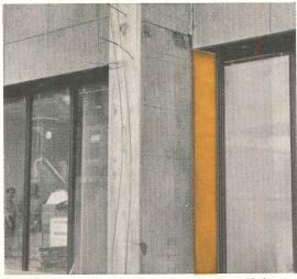
UPRIGHT CONCRETE GIRDER before covering with bronze "skin." The Revere Muntz Metal used was in thicknesses of 1/8" and 3/16", ranging up to 40" in width by 11' 11" in length.
