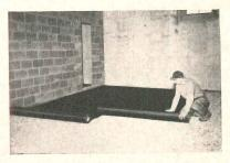
**SISALKRAFT,** tough, reinforced waterproof papers for protecting floors, curing concrete, covering unfinished work on the job. In fact, any application requiring protection against the weather.
