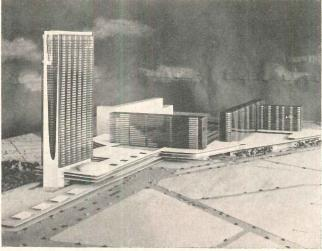
Railroad station is on lower floors of tower. Long station structure will continue at same height to form wings for other buildings, none less than 18 stories high. Tracks will be roofed over. Underneath buildings and triangular esplanade, planted with trees and shrubs will be railroad installations and parking area
