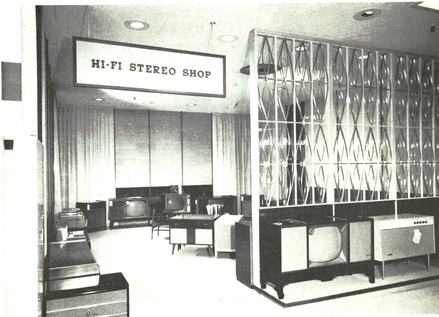
A decorative metal grill separates and defines the Hi-Fi and television department as a small shop
