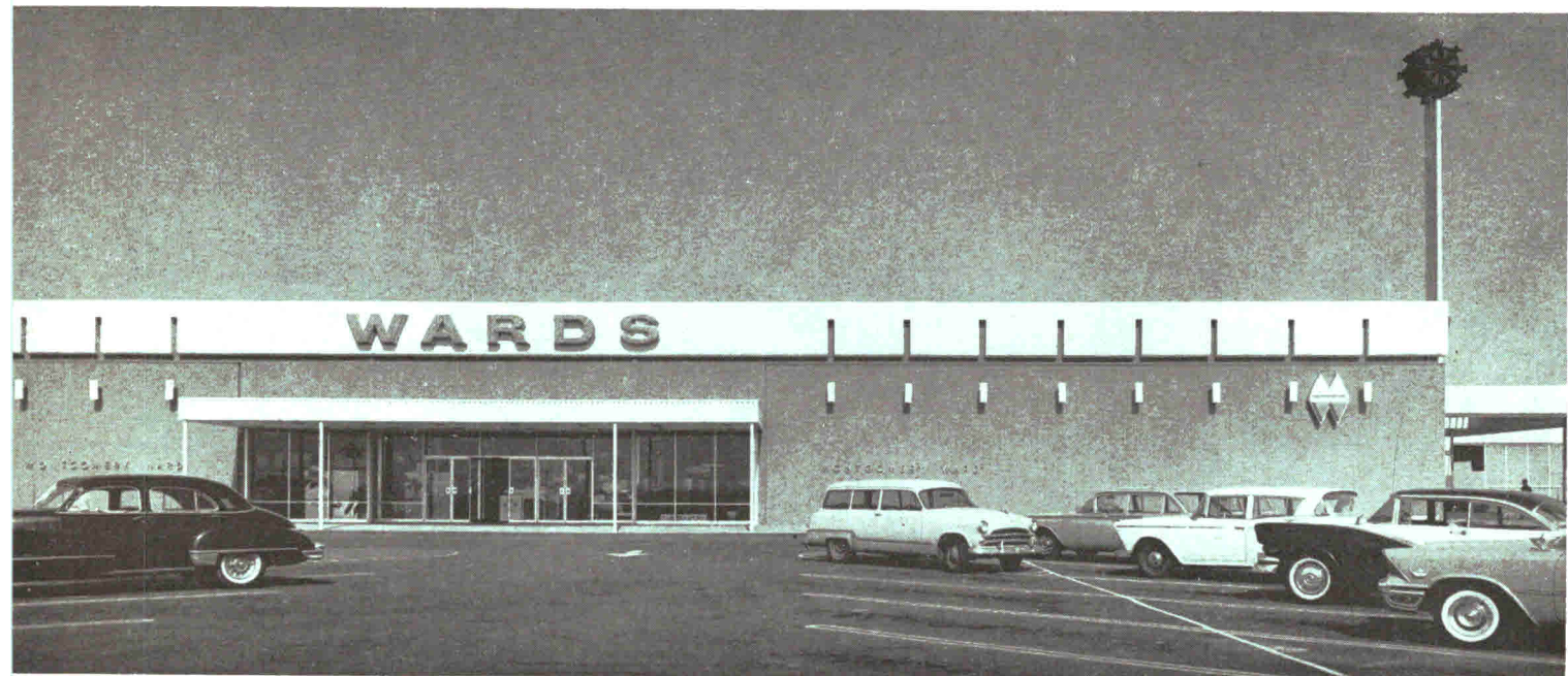
Montgomery Ward store has concrete block walls, plaster fascia, metal canopy. Exterior lights make pattern on wall
