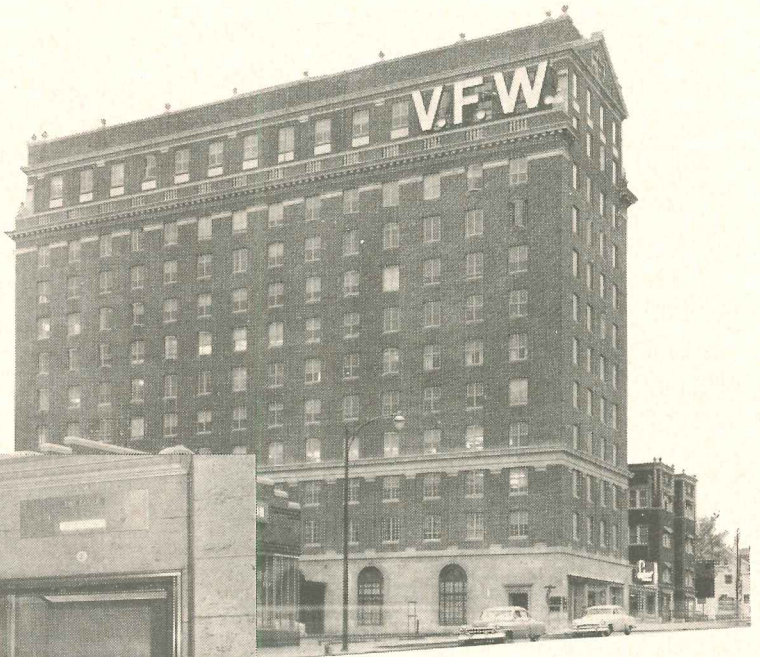
VFW BUILDING, KANSAS CITY, MISSOURI
