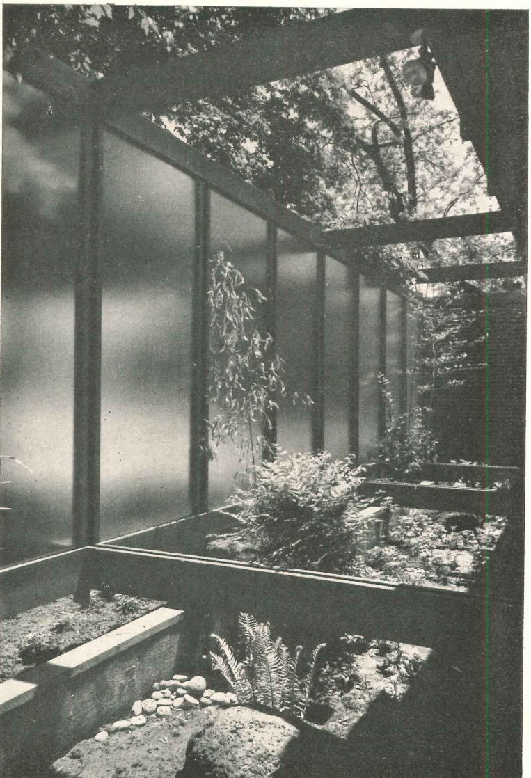
Far-reaching double-plank beams and supports of wood frame the translucent glass panels around an informal garden, let the outdoors in naturally for a relaxed atmosphere throughout the clinic.
