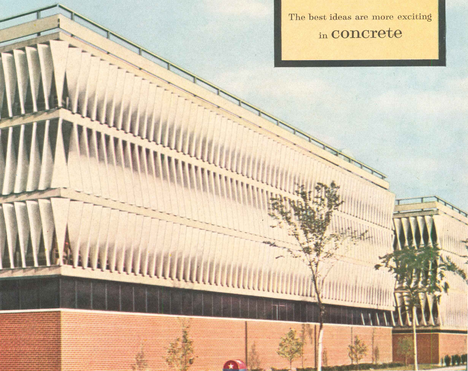
Henry Ford Hospital 870-car parking structure, Detroit, Michigan. Architect: Albert Kahn, Associated Architects and Engineers, Inc., Detroit, Michigan
