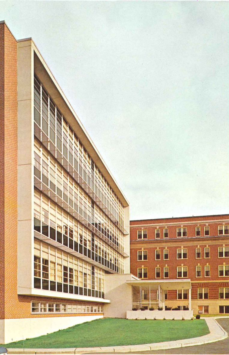
Sweeping glass façade in the new wing of Roger Williams General Hospital, Providence, R.I. Architects: Howe & Prout, Providence. L·O·F Vitrolux was used in the spandrels, Thermopane in the windows.
