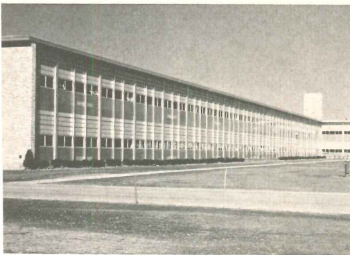
Architect Enos Cooke, New Kensington, Pa., used Thinlite in a major way at Stewart Junior High School, Lower Burrell Township, Pa., blending light-controlling panels with windows and aluminum-faced insulating panels.
