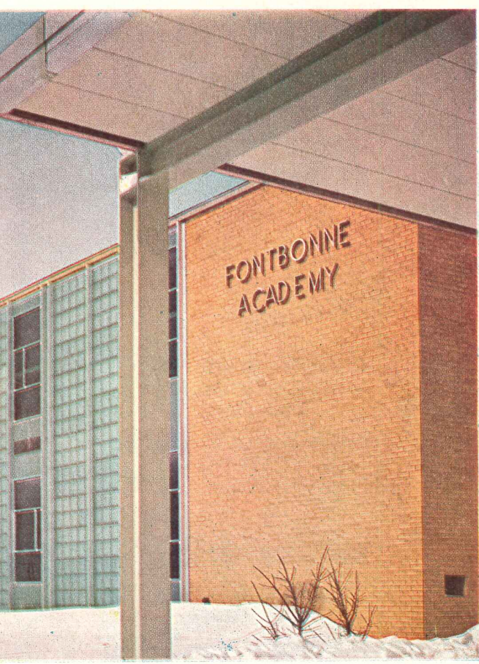
At Fontbonne Academy, Allegheny County, Pa., architects Celli-Flynn, McKeesport, combined light-controlling panels of green Thinlite with window and metal panels to achieve this unusual effect in the classroom wing.
