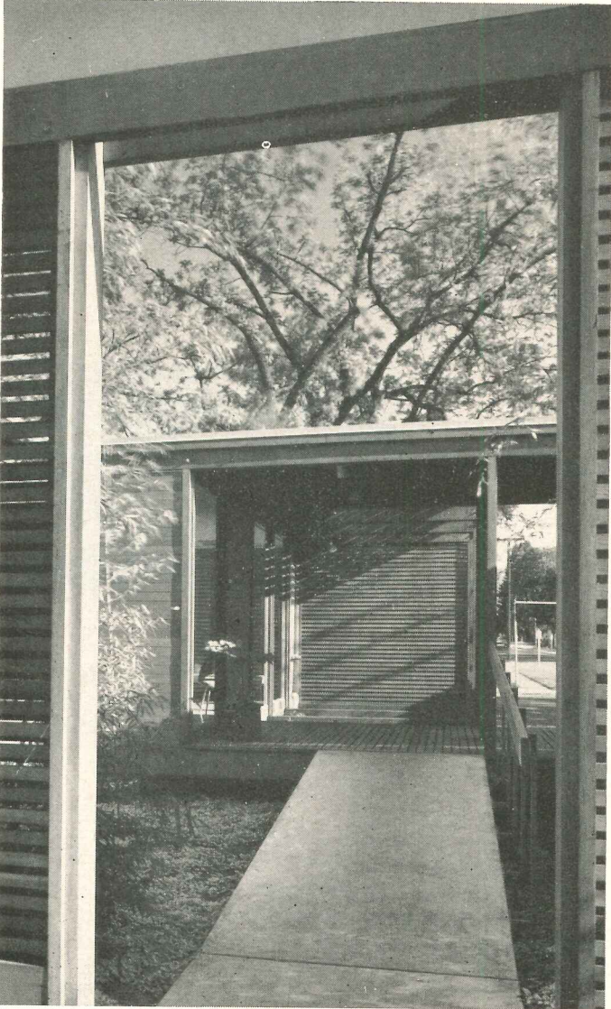
Wood bares still more of its friendliness in the dental clinic's intimate courtyard. The wall of spaced siding offers ample privacy with open-air freedom, clearly demonstrates one of wood's many economies.
