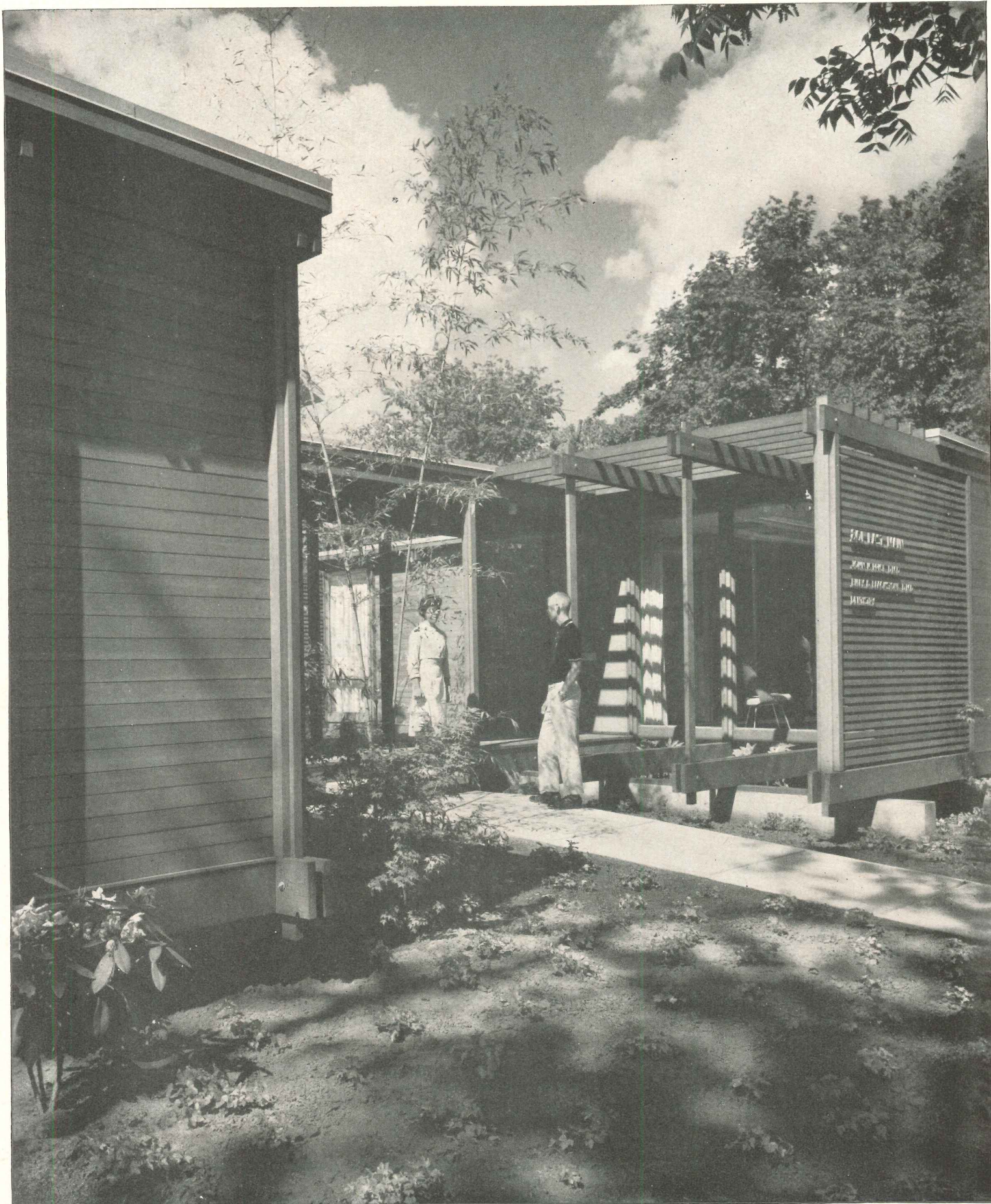
A unique dental clinic attests best to wood's natural adaptability and warmth. The simplicity of exposed beams and supports bolted together, the mixture of spaced and solid siding complementing one another—all present a friendly outside, promise a comfortable inside. Architects: Kirk, Wallace, McKinley & Assoc., A.I.A.
