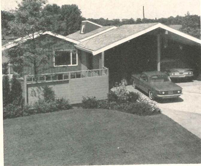
Architects: Bassetti & Morse, Seattle. Location: North Canton, Ohio. Builder: J. R. Wilkin, in cooperation with the Ohio Power Company
