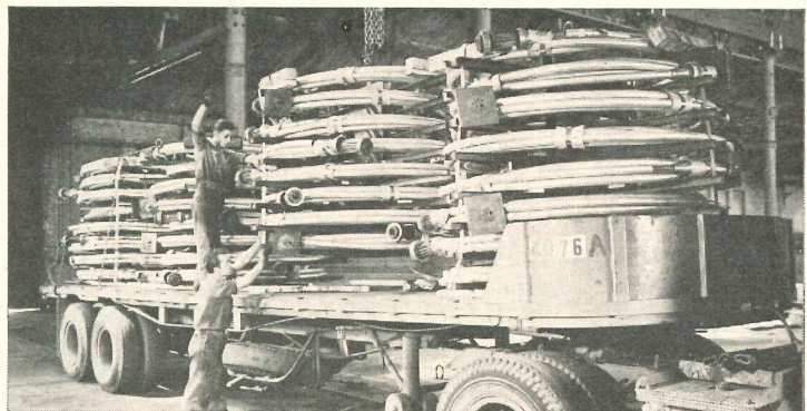
Completely Assembled Tendons —are shipped on specially designed incoiling racks ready for easy installation.
