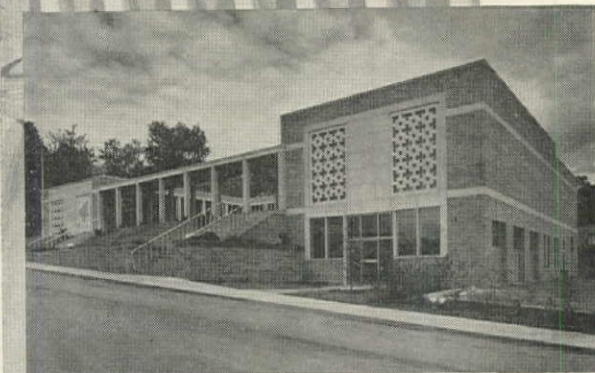
GREENEVILLE LIGHT & POWER BLDG., Greenville, Tenn. Architect: Honeycutt & Boyd, Greenville, Tenn. Gen. Contractor: Hogan Bros., Greenville, Tenn. Panels by Southern Cast Stone Co., Knoxville, Tenn.
