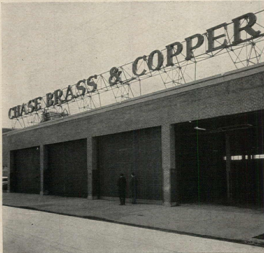
Chase Brass & Copper Co. Long Island Warehouse Arch./Engr.—Lockwood-Greene Engrs., Inc. Contr.—Gilbane Building Co.
