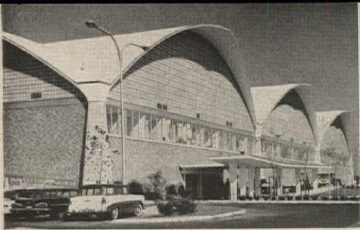
Light-controlling Thinlite panels provide excellent natural light, help reduce heating and cooling costs for the new $20-million Intelix Systems Post Office in Providence, R. I. Charles A. Maguire & Assoc., Providence, supervised design and construction.
