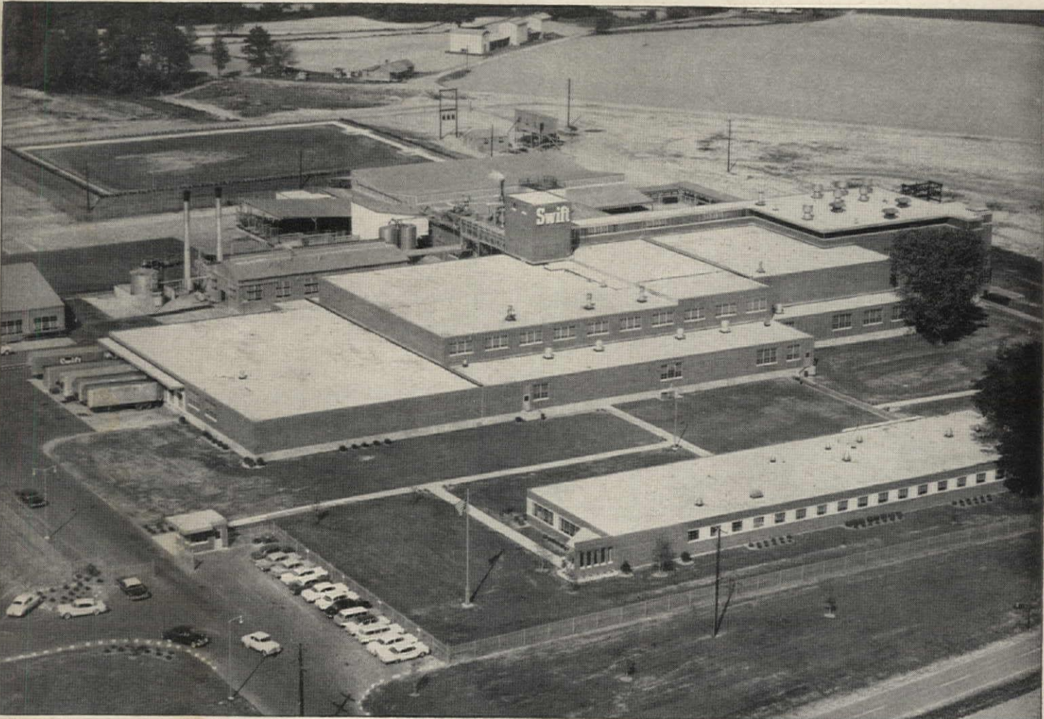
Swift and Company Packing Plant, Wilson, North Carolina. ARCHITECT: Swift and Co. Staff. CONTRACTOR: F. N. Thompson, Inc.
