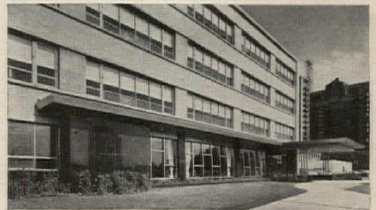
Fantus Outpatient Clinic, Chicago ARCHITECTS: Richard W. Prendergast & Associates CONTRACTOR: Mayfair Construction Co. STAINLESS STEEL WINDOW MFR.: Flour City Architectural Metals Division, Hupp Corporation
