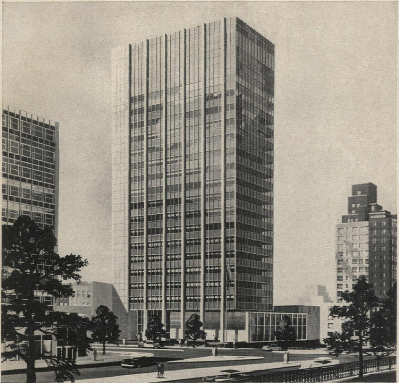
LIFETIME GOOD LOOKS — Scheduled for completion by mid-1961, New York's United Engineering Center will provide 260,000 square feet gross area for 18 engineering bodies. Exterior of Nickel Stainless Steel
