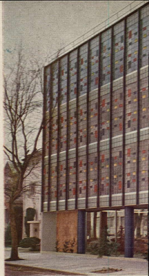
Thinlite panels of Clear Vista, accented with ceramic colors, add maximum light with low heat transmission in the new office building of the State Employees Building Corp., Sacramento, Calif. West American Engineering Co., Inc., San Francisco, designed the structure.
