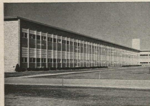
Architect Enos Cooke, New Kensington, Pa., used Thinlite in a major way at Stewart Junior High School, Lower Burrell Township, Pa., blending light-controlling panels with windows and aluminum-faced insulating panels.
