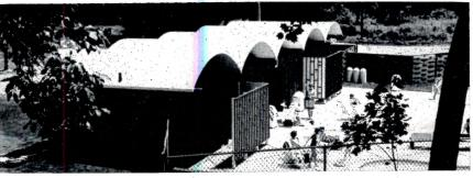
Weatherproofing of roofs of any concour, such as curved shells, folded plates and hyperbolic paraboloids, as well as domes and flat roofs, is possible with a one-ply built-up roofing system which can be used on any nailable or non-nailable flat or steep goof deck.
