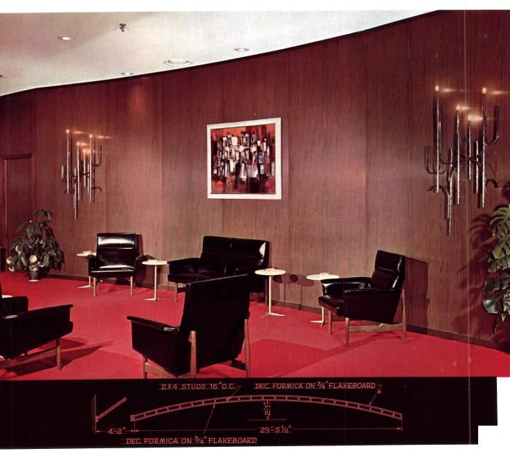
A decorative non-loadbearing wall can be erected quickly and inexpensively to any shape with Formica laminated plastic.
