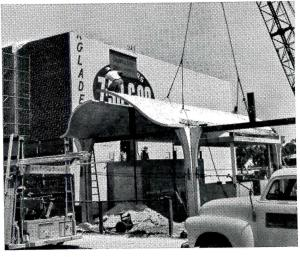
(Above) With precast columns in place, half-shells are set with minimum difficulty. Note the temporary edge beam and vertical supports which were removed as each completed pair of shells took up the load. Shell units are 48' long, 8' wide, 3" thick and weigh 7 tons each. The precast columns are 44" wide at the top, 16" wide at the bottom. Each is 11'9" long.
