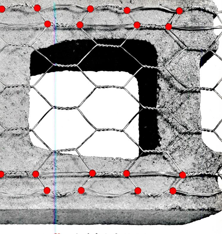
28 mortar locks to the block foot with Keywall reinforcement. The more locks, the more resistance to cracks resulting from shrinkage. Movement is restrained at each of Keywall's mortar locks. No one lock has to restrain more than the movement in 3/4" of block. That's the kind of reinforcement that works.
