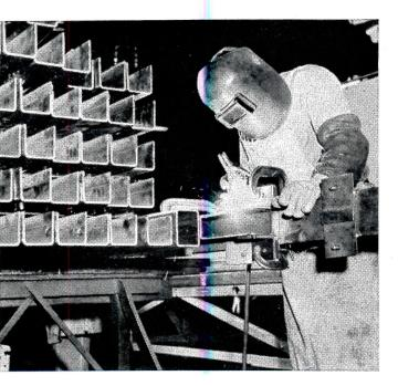
**OFF-SITE FABRICATION:** Welding heavy steel angles for structural steel anchoring to both sides and ends of Republic Rectangular Steel Tubing. Tubing used at New York Life Insurance Company's new headquarters in New York City. Tubing fabricated by General Bronze Corporation, Garden City, Long Island, N. Y.
