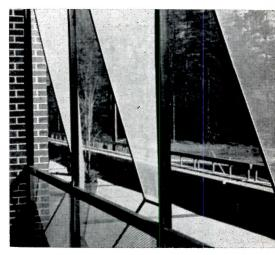
A uniformly textured façade for apartment buildings with balconies provided by screens of *Fiberglas* cloth, held in aluminum frames to form any desired pattern.
