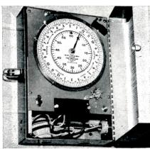
One program clock actuates series of G-E motorized controls which switch thousands of lamps ON or OFF, through low-voltage circuits and relays.
