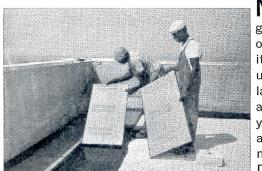
Nothing but FOAMGLAS Roof Insulation gives a building the constant insulating value that results from an inorganic, cellular glass composition. It just can't absorb moisture. And, it's available now in a 1½" thick FOAMGLAS-BOARD PITTSBURGH unit—a sandwich of FOAMGLAS covered with kraft
