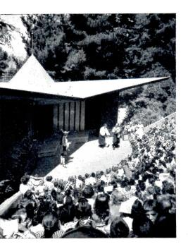
THIS INGENIOUS STAR-SHAPED ROOF demonstrates the remarkable structural forms that can be achieved with plywood. Deceptively simple, the design bears more resemblance to airplane wings than a conventional roof, with interacting plywood and lightweight lumber members forming skeleton and structural skin.
