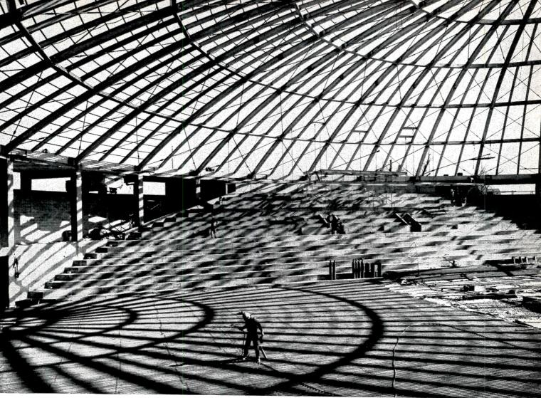
The Brown rink during construction. The steel pipe was laid on 4-in. centers, tested out at 100 psi, then buried in 15%-in. of concrete. Henry J. Coupe & Son, Inc., did the refrigeration and piping work. The Bethlehem steel pipe was supplied by United Supply Co.
