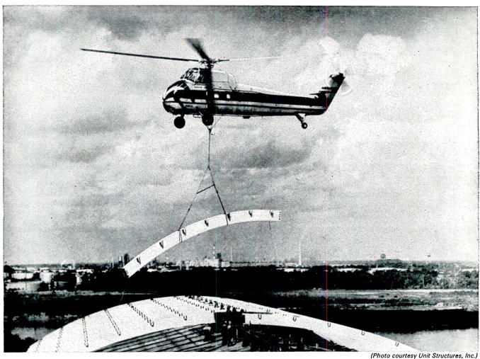
Helicopter lowers structural section of laminated SPA Southern Pine into new roof system of large chemical plant. This efficient operation saved days of construction time, resulted in substantial savings.
