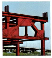
Steel trusses support Constitution Plaza's Americana Hotel over a city street. They were erected by National Steel Fabricators, Inc., and fabricated by Bethlehem Fabricators, Inc. Bethlehem steel bars also reinforce the structure's concrete work.
