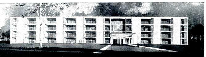
NURSING CARE BUILDING, Lyngblomsten Retirement Center, St. Paul, Minn., uses Ryerson post-tensioning to maximize the economies and efficiencies of lift-slab construction, and provide deflection control. Four-story structure has 2 lift-slabs (connected by a joining strip after lifting) on each of 5 levels. Each two-unit slab measures approx-
