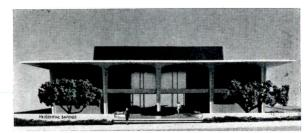
BRANCH BANK: This two-story building for Prudential Savings and Loan Company in Alhambra, Calif., is of concrete and brick filler panels. Structural concrete columns, handsomely shaped, support a flat plate concrete roof; inside, the ceiling of the banking room is slightly vaulted, and is daylighted by a large central skylight. A mezzanine work area around three sides of the banking room provides public meeting facilities and office space. Architects: Ladd & Kelsey
