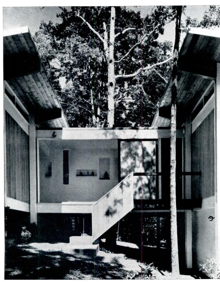
A wooded background naturally suits the extensive use of wood in this home's siding, overhanging roof, and exposed framing. See, too, how different forms of wood attractively complement one another, as in the solid stair-railing and open-rail entranceway.
