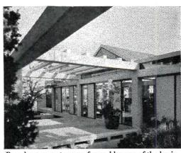
Broad entrance terrace, formed by one of the basic "Space Frame" units. Floor is of 2' x 16' precast concrete panels.
