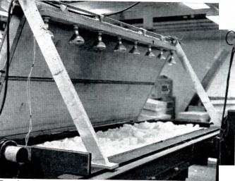
Dry ice, 3 to 4 in. deep, dumped on top of the test specimendrops the temperature of roofing all the way down to -100 F
