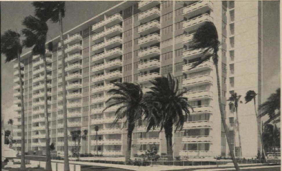
Point View North is a 13-story structure with reinforced concrete frame, floors and roof, with concrete masonry stuccoed walls. Owner: Paul Dennis, New York City. Architect: Charles F. McKirahan & Associates, Ft. Lauderdale. Structural Engineer: D. E. Britt & Associates, Miami Beach. General Contractor: Frank J. Rooney, Inc., Miami. Plastering Contractor: John W. Thomson & Son, Inc., Miami.
