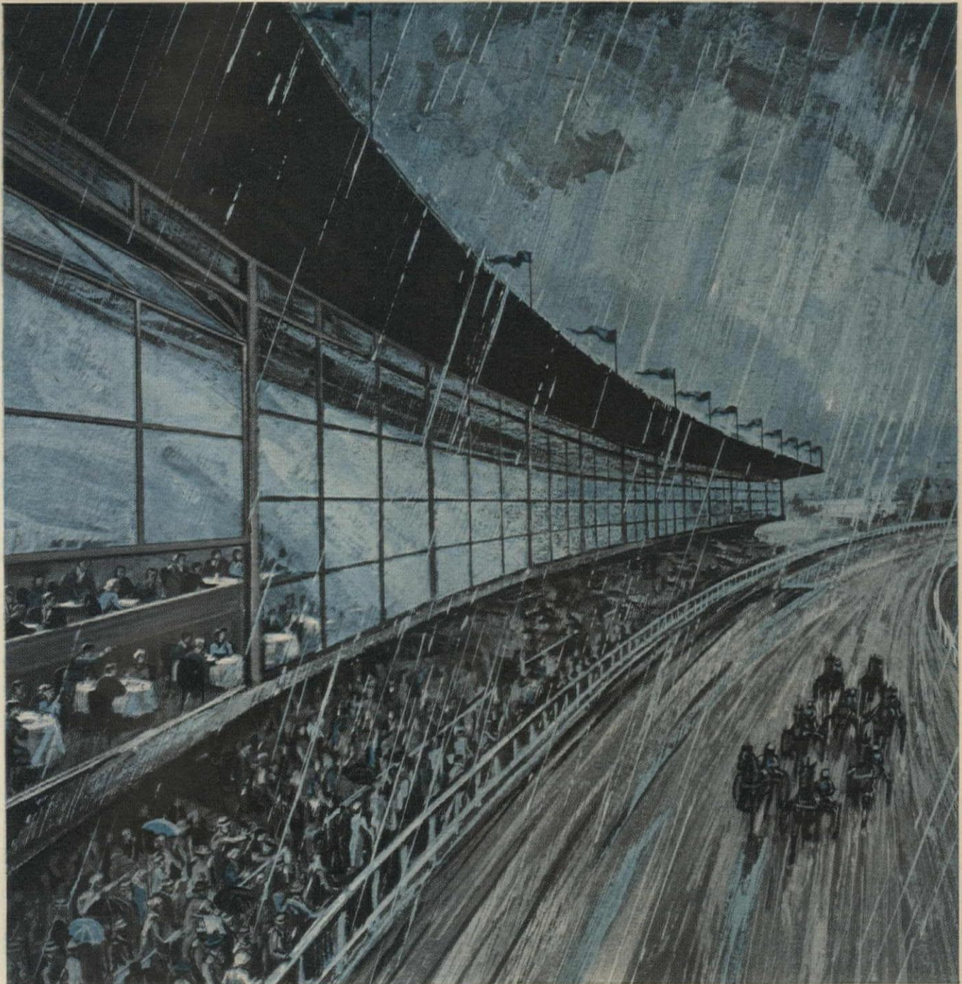
Panoramic aluminum "OVERHEAD DOORS" at Vernon Downs Racetrack, Vernon, New York
