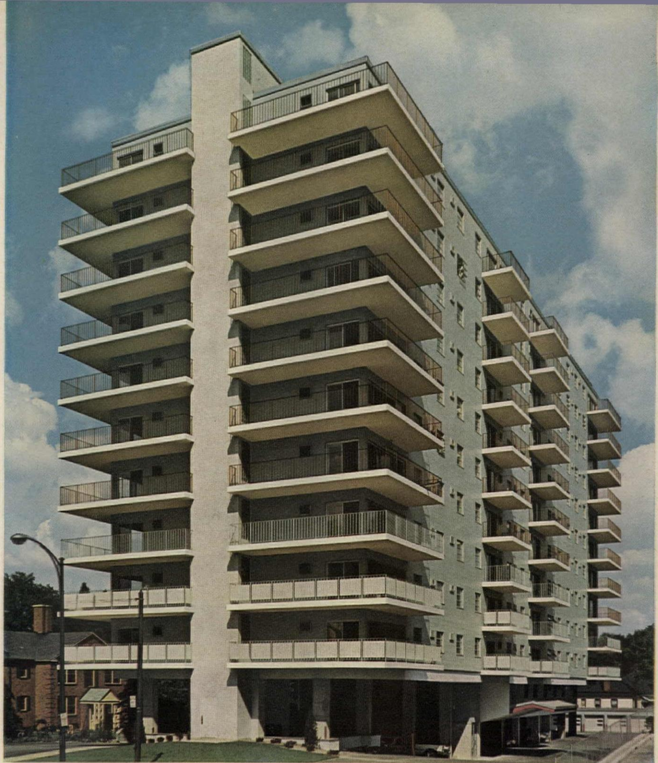
1217 Delaware Avenue Apartments, Buffalo, N.Y. Owner-Builder: BCH Construction Corporation.
