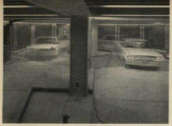
Installation of a hollow turntable around an existing building column provides drive-in facilities in a bank in Minneapolis.
