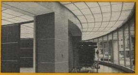
Tee system designed to conform with circular building shape and coordinated with structural steel and ductwork to provide flexibility for partition layout.
