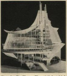
French Pavilion: The 140-foot-high French Pavilion will have a steel framework covered with glass and aluminum. The \$4 million structure will have exhibits on seven levels above a water cascade and garden. Architect is J. Faugeron and André Blouin is Canadian associate.
