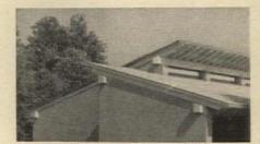
The basic structural vocabulary of all the campus buildings consists of pitched roofs, overhanging eaves and clerestories. The roof structure is clearly expressed without and within. Bearing walls and columns are of salmon-colored brick. For all buildings the column module was kept as consistent as possible within the plan requirements.
