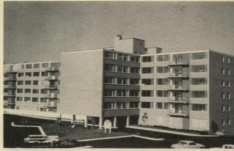
The Madison Apartment uses a practically uniform bay spacing in each wing. The joist and structural steel weight, including columns, was only 6 lb per sq ft and the erected price of steel was \$108,950, or 90 cents per sq ft.
