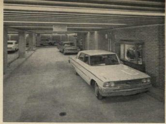
Tellers booths are on the exit side of the turntable; an automatic gate closes the turntable if all three booths are occupied.
