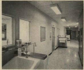
Nursing stations contain medicine preparation areas and are adjacent to doctors' charting rooms with provision of a horizontally slotted pass-through chart rack which improves doctors' visual privacy while maintaining needed chart interchange and vocal contact. Clean supplies are delivered to one side of a vertically divided pass-through closet at each patient room. Soiled supplies are periodically removed through the other side of this closet (bottom, right).
