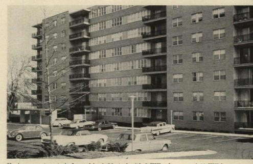
Horizon apartments is framed in A-36 steel with 8 WF columns and 10 WF beams. Uniform bay sizes were used for framing, but modified by offsetting end bays, producing a slight variation in plan and breaking up an otherwise flat facade.
