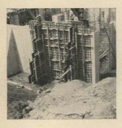
The necessity for completing the new, 51,500 seat Atlanta Municipal Stadium in less than one year dictated the use of Symons Steel-Ply Gang Forms for column, outer bearing wall and buttress forming, according to the contractor, Thompson Street Company, Charlotte, North Carolina.
