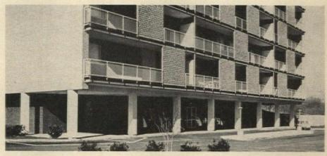
Regular bay spacing is essenial to economical welded framing, above. Balconies can be supported by cantilevered rectangular tubes (with drain holes), below.
