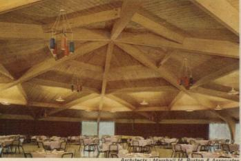
re-shrunk to full American Lumber Standard sizes, Southren Pine provides stability and precision essential to engieered construction, as in this country club. Standard grades an be utilized for cantilevered and continuous members ithout special grading.
