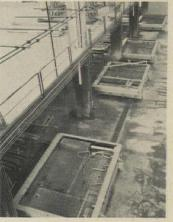
At the factory, interior partitions are poured vertically, with the concrete being introduced at the bottom of the form to avoid air pockets. Heating of forms enables panels to be produced at rate of one every three hours. Battery of 11 casting machines produces 10,000 sq ft of load-bearing walls per day. Exterior wall panels are poured horizontally, in order to introduce exterior finish and insulation (right). Interior partitions containing plumbing are also poured flat (left).
