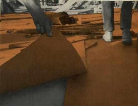
Sisalkraft Reinforced Paper is 5-plies strong, so it protects the surface against abrasion and soiling from traffic and debris, and reduces clean-up costs. Sisalkraft is also waterproof, prolonging the hydration process to produce a denser, more uniformly cured slab.
