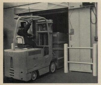
Trucks move in and out of  $-10^{\circ}$ F. temperature without delay. Electroglide doors—with remote control operation—close at 1.5 fps to reduce loss of cold air.
