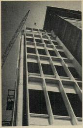
A complete production line was set up on the site of the nine-story Alameda Building in San Jose, California for precasting walls, girders, and pretensioned slabs. Columns, spandrel beams and slab topping were poured in place, and the core was slip-formed. A tower crane, moving on rails, handled precast components and hoisted concrete for *in-situ* operations. Architect: Allan M. Water & Associates; structural engineers: T. Y. Lin, Kulka, Yang and Associates.
