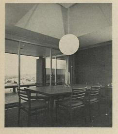
it, "permits interior space to be molded by simply turning up the ceiling between the trusses to produce high ceilings where desired." These high ceilings rise in the form of truncated pyramids over the living room, gallery and the four corner rooms, and are capped by light diffusing skylights. Spherical light fixtures are suspended in some of these recesses.
