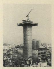
Suspension system uses a central mechanical core from which floors are hung—beginning from the top. Shown is the 23-story Kleinwort-Benson building in London.
