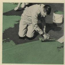
Quick, easy application. Just prime the surface, add catalyst to Traffic Topping, mix and trowel on. No expensive equipment needed. Only one coat is usually required, so application costs are low.
