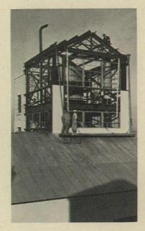
It's a panel of Hetrofoam®-based polyurethane foam between asbestoscement sheeting, developed by National Gypsum Company.
