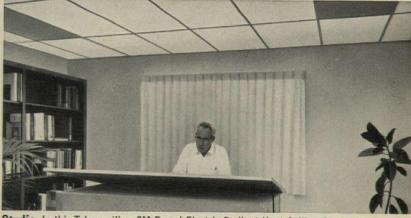
Studio. In this T-bar ceiling, 3M Brand Electric Radiant Heat Ceiling Panels (the opaque ones) blend with the illuminated panels. They provide warmth in soft, gentle rays. No drafts. No noise—not even a whisper. No wasted space. 2'x 4' drop-in panels (500 watts).
