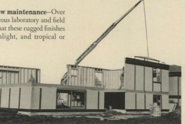
Wall section for this new house is lifted by boom crane and moved into position for installation. Interior wall is completed with foil-faced fiber insulation and ½ in. dry walls. Prefabricated walls are erected quickly and easily.
