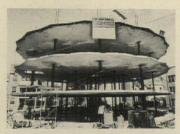
Lift-slab construction has provided about a decade of demonstration of economy in ground-level fabrication. Shown is St. John's nursing home in Milwaukee, Charles Haeuser, architect.
