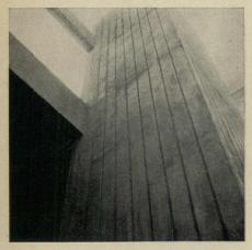
Two 3-story concrete towers, unbroken by windows or other openings, will provide the passerby with an attractive view due to a pleasing architectural treatment of the walls. The job is in Norwalk, Connecticut, by contractor Thomas H. Riordan. The building itself is roughly "T" shaped, and the architectural walls are on the elevator and utility cores of the new structure.
