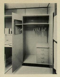
developed for installation in educational institutions. The rooms consist of acoustical-paneled walls with steel skins and foam plastic core, acoustical tile ceilings, including fluorescent lighting with air diffusing devices and floors of asphalt tile. Variations of the design may be obtained as well as different combinations of built-in and movable furniture.
