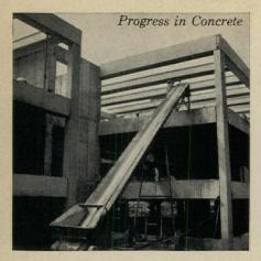
ARCHITECTURAL FORMING WITH SYMONS STEEL-PLY PANELS AND V-SHAPED CHAMFER STRIPS
