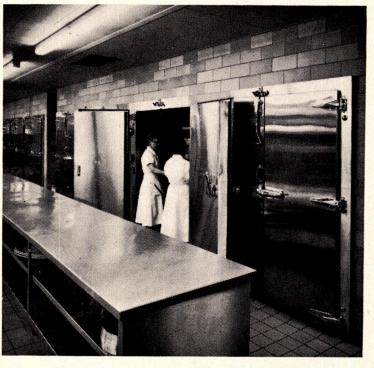
Jamison FS double cooler and freezer doors in hotel kitchen are completely stainless clad for easy cleaning and bright appearance.
