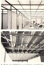
A first in lighting-cooling-partitioning flexibility was the ceiling of SOM's Union Carbide Building, for which Syska & Hennessy were consulting mechanical and electrical engineers. This system of continuous fixtures marked by a grid which functions for both air supply and partition anchoring was fully described in the February 1960 RECORD.
