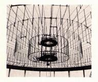
A great deal of engineering sophistication is built into the modern cable roof. In the example above loads are carried to the ground by a lightweight X-frame which also prevents bending in the compression ring when there are unbalanced loads. The Oakland-Alameda Coliseum by Skidmore, Owings & Merrill, San Francisco: roof consultant, Ammann & Whitney, Struts in the cable roof, left, together
