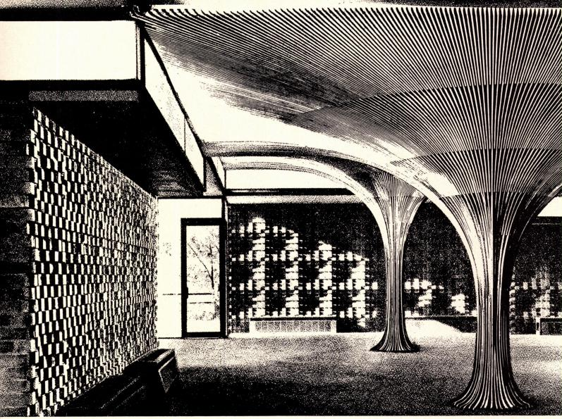
Plastic forms were used for precision casting of these columns. The high-early-strength concrete, made with Lone Star's INCOR® 24-hour portland cement, permitted forms to be stripped the following day. Maximum aggregate size was 3/s".
