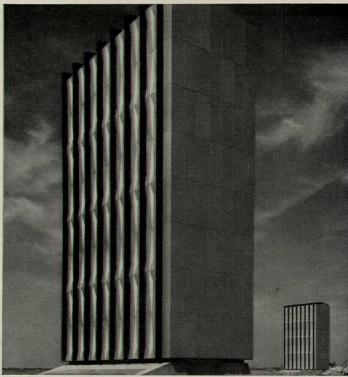
Corrosion Resistance—These intake gate structures, each nearly 100 feet high, are clad with matte-finished stainless steel panels for strength and stability in a corrosive environment. Niagara Power Project, Niagara Falls, N.Y. Engineers and Designers: Uhl, Hall and Rich, Boston, Mass. Architectural Consultant: John B. Peterkin, New York, N.Y. Stainless steel panels: General Bronze Corp., New York, N.Y.
