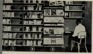
1. Fold-a-Shelves. Meet every strength specification yet fold down for easy storage. Brackets remain vertical when adjusting. 2. Divided Shelves. 3. Sloping Periodical Shelves, hinged to provide easy access to stored publications. 4. Light-weight desk with Bracket Shelving above.
