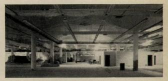
42-ft.-sq. column-free bays, required by Monarch for their many and varied production activities, provide a high degree of interior flexibility. Equipment and people can be freely shifted to accommodate new improved work flow patterns as they are developed. With the umbrella HP roof, 60-ft.-square bays are not uncommon.
