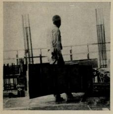
When Henry C. Beck Co. exceeded original cost estimates on a 20-story La Jolla, California, high rise, it decided to use Symons Slab Shore system in an effort to cancel the loss. Initial loss was recovered, and scheduled per floor construction time was reduced from 5 to 4 days.
