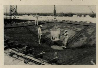
Through use of 4,000 psi high-early-strength concrete, shells were concreted at a 2-per-day rate. Before form removal, specifications required a strength of 3,200 psi, which occurred in 36 to 40 hours with the following mix proportions: Type III cement, 564 lb.; water, 267 lb.; sand, 1,300 lb.; <sup>3</sup>/<sub>4</sub>-in. aggregate, 1,890 lb.; entrained air, 6 percent.
