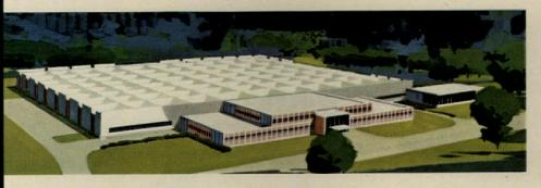
The new office-plant structure of the Monarch Marking System Company near Dayton, Ohio, demonstrates the excitement concrete can bring to industrial buildings. To cover the plant area, architects created a single 3½-acre roof by joining 88 inverted concrete umbrellas 42 feet square, each one self-supporting.
