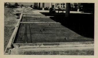
6-in. wall panels, each 26 ft. tall and 19 ft. wide, were conveniently cast right on the plant floor adjacent to their final positions in the wall. When tilted into place, the under side of the panel became the inside face of the wall. The top side, simply screeded and troweled, became the exterior face. 3,000 psi ready mixed concrete of the following mix proportions was used: Type I cement, 470 lb.; water, 240 lb.; sand, 1,465 lb.; 3/4-in. aggregate, 1,921 lb.; entrained air, 5 percent.
