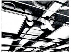
Air distribution is by a dual-duct system. From the mixing boxes located in each zone, air goes to air diffusers mounted on the sides of the troffers. At present only half of the troffers are used to either supply or exhaust air. If necessary, present connections can be shifted to suit a new partitioning arrangement.
