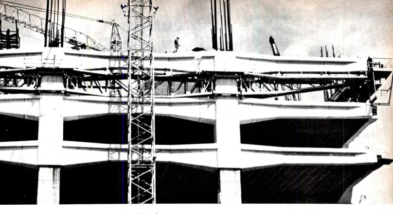
elevators. In addition to serving as the interior support for the precast floor framing system, the core resists all of the wind forces on the building.
