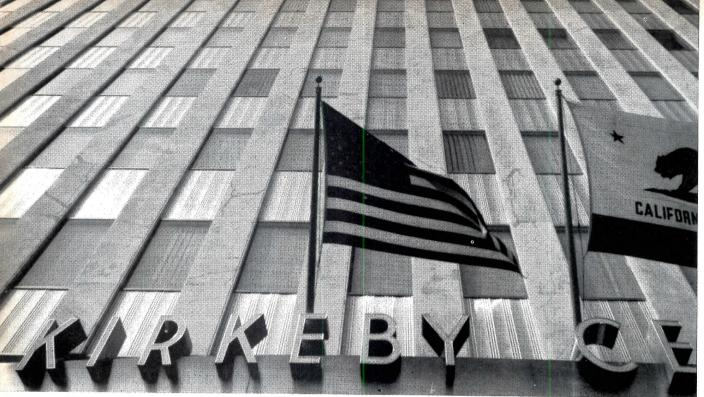
LUSTROUS stainless steel spandrels with No. 4 finish alternate with white marble piers at Kirkeby Center, Los Angeles, California. Architects: Claud Beelman and Associates, Los Angeles, Cal. Spandrels, fluted to provide stiffness and eliminate optical distortion, by Construction Metalwork Corp., El Monte, Cal.
