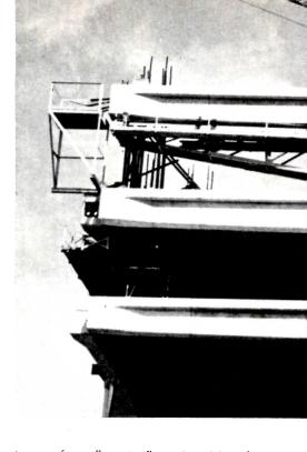
An architectural requirement was that the inner face of the exterior frame elements—that is columns and beams—should be in the same plane, permitting a continuous glass line inside the structural frame.
