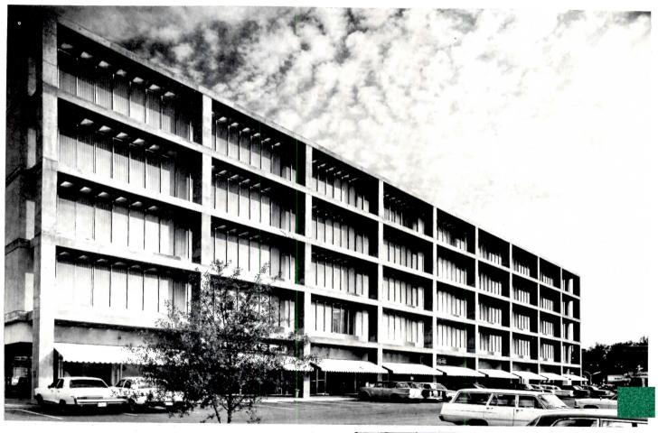
This speculative office building, located in a landscape that consists mostly of parking lots, has a strong simple form that is well adapted to its size and the needs of its tenants. The bays are on 27-foot centers; the over-all length from end of stair towers is 284 feet; the width is 72 feet over-all.
