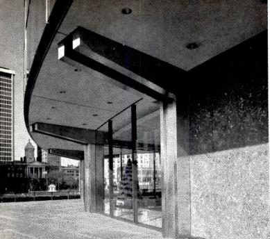
MIRROR FINISHED stainless steel accents red marble and blast-finished granite and provides durability with minimum maintenance in the Sun Life Building, Baltimore, Md. Architect: Peterson and Brickbauer, Baltimore, in association with Emery Roth & Sons. Stainless steel entrances, column covers and window framing: Allied-Superb Bronze Corp., New York, N. Y.
