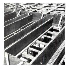
Gunnar I. Johnson, Minnesota contractor on the 4 story Science Hall at St. John's University, used a unique pan and joist construction shoring method to support 24" deep, 8½" wide joists. Joists were 4' c.c., and shoring had to be held exactly to these dimensions.
