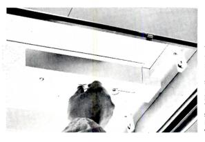
To change from a two-lamp to a four-lamp fixture it is necessary only to snap open the lens, shorten the special telescoping wiring channel, and unlock the wing bolts which hold the channel in the troffer. The entire channel, containing sockets, ballasts and wiring, is held by a chain while the workman unhooks wiring.
