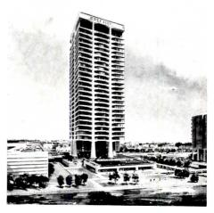
There is increasing evidence that architects and engineers are finally taking more advantage of the esthetic, structural and construction potentialities of precast concrete. Case in point: the design of the new 27-story Gulf Life Insurance Company building in Jacksonville, Florida, said to be the nation's tallest precast, segmented, post-tensioned building. It was designed by Welton Becket and Associates, architects and engineers, with Richard Bradshaw as structural engineer.
