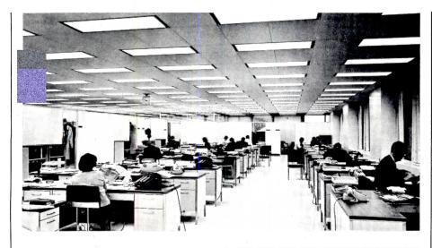
Combination lighting, airhandling troffers in the new 31-story Illinois Bell Telephone office building can easily be changed from two-lamp fixtures to four-lamp fixtures, raising the footcandle level from 85 to approximately 150. Similarly, the air-handling unit can be adjusted to deliver from 50 to 120 cfm of tempered air.
