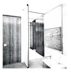
MOVABLE WALLS / A system that can be installed in schools, restaurants, offices and other heavy traffic public areas provides an acoustically-sealed flat wall that can be readily moved by custodial help to suit changing requirements. Mechanically expanded rubber shoes press against the floor and ceiling to close the opening. No floor track is required.
