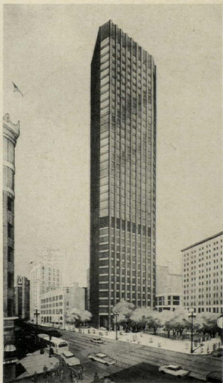
A 38-story office building in San Francisco, designed by Welton Becket and Associates, will have 3-foot 10-inch square columns, sheathed in dark stone, rising the height of the building. The building, covering less than 55 per cent of the site, will be located in a landscaped stone plaza with a sunken plaza entrance to a rapid transit station. The building will replace the old Crocker Building, built in 1892. Landscape architect is Sasaki, Walker Associates and contractor will be the Dinwiddie Construction Company.
