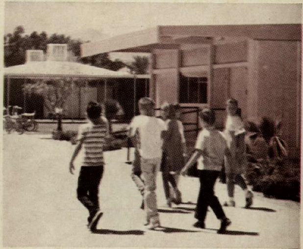
These children will be middle-aged before the 40-year minimum life expectancy of these mobile school buildings expires. A wall core of rigid urethane foam combines structural strength and insulation for long-term economies.
