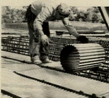
Deck can be easily placed by one man.
