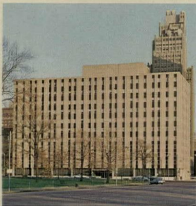
Southwestern Bell Telephone Office Building
