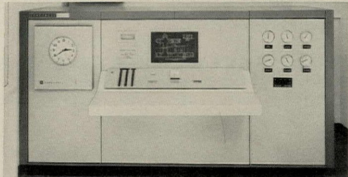
Honeywell Selectograph displays and controls functioning of air-handling systems.
