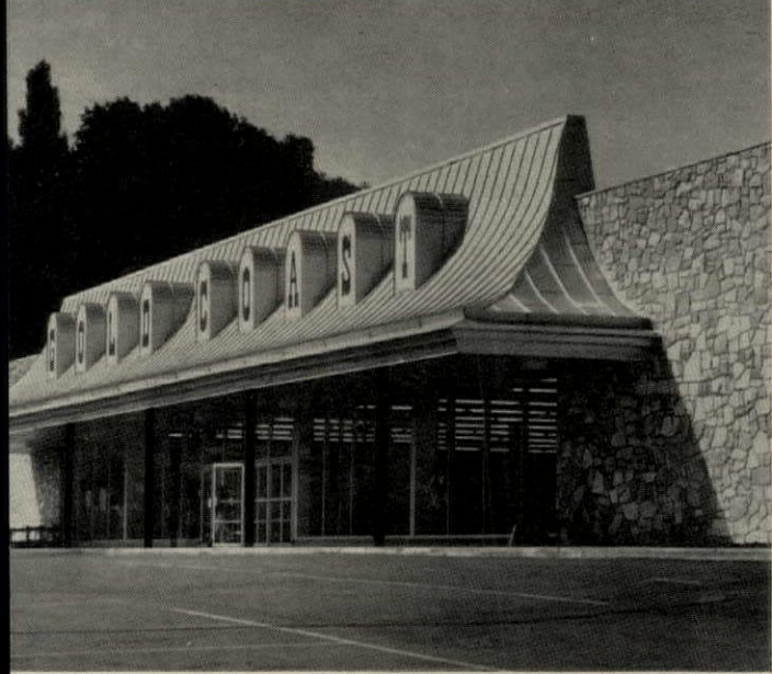
STAINLESS STEEL standing seam roof, valley flashing, fascia, gutters and downspouts. The Gold Coast, Maitland, Pa. Architect: Lucian Castiglione. General Contractor: Castle Development Co. Roofing Contractor: General Roofing Co.
