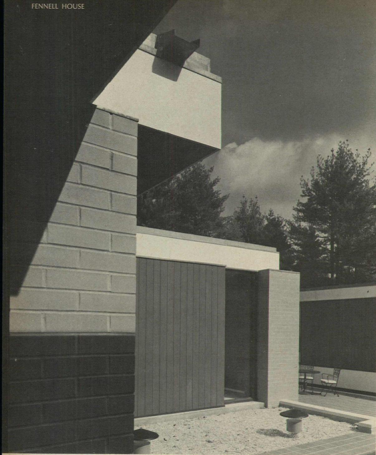
The modular construction system uses brick columns with steel-beam framing and wood joists spanning between beams. The constant roof line creates a strong white fascia effect all around the house, giving unity to the building as a whole. The roof line is set back from the edge of the masonry columns. Exterior walls are vertical cedar boards, redwood trim and areas of glass.
