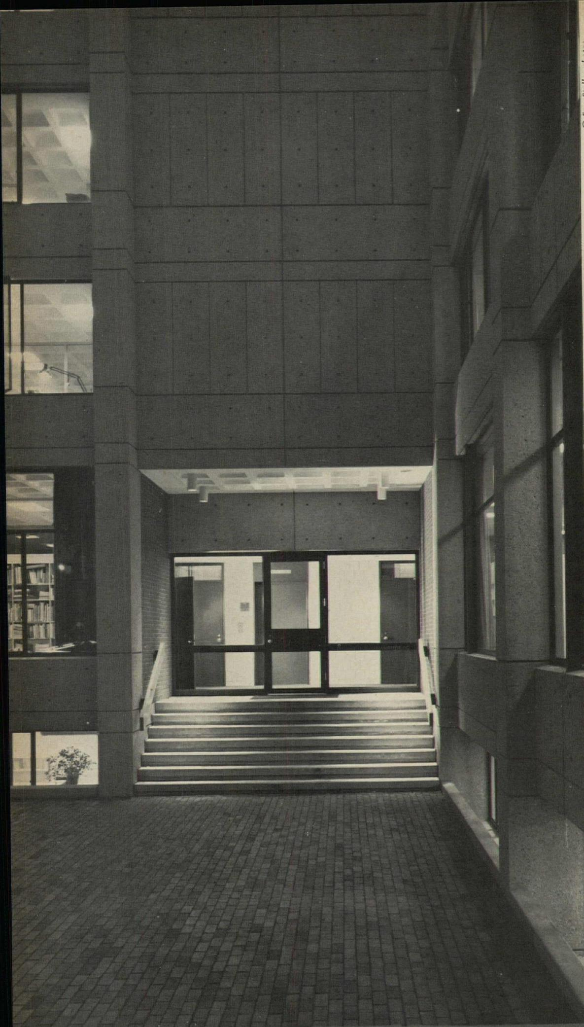
**Enrichment of the concrete surface** has been achieved by simple means. Holes left by the wooden lags and the formwork combine with the raked joints to form a handsome, well-scaled pattern as shown in the photograph at left. The sandblasted surface reveals an attractive aggregate of dark gravel which contrasts well with the bronze colored glass of the windows. Sidewalks and the courtyard are also of brick.
