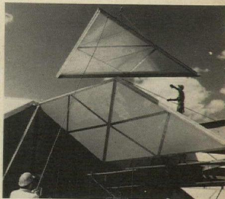
Austrian pavilion's large modular structural units are made up of four separate panels. Each panel is filled with Union Camp kraft Honeycomb cores. These give facings continuous support—eliminate need for rivets or spot welds that have to be finished off before painting.
