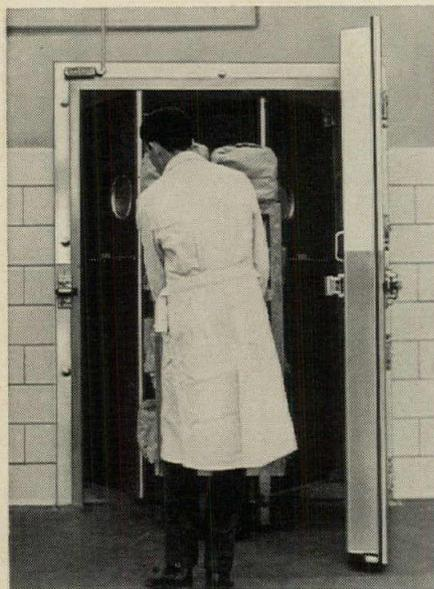
▲ JAMOTUF® freezer door installed in extra wide doorway for passage of hand trucks. Door is equipped with Frostop® heater cables to prevent icing of gasket contact areas. 16 gauge stainless steel "kick plate" protects door against impact and abuse.
