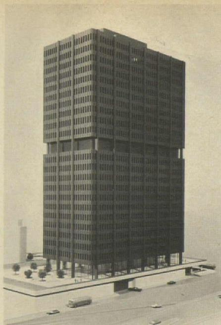
The Westinghouse Building in Gateway Center, Pittsburgh, designed by Harrison and Abramovitz and owned and operated by The Equitable Life Assurance Society of the U.S., will be a 23-story office building of steel-frame construction with cellular steel floor decks. The building, which will contain 500,000 square feet, will have an all-electric system, with the heat from the lighting system utilized for needs within the building.
