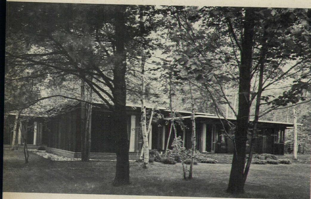
**Dow:** This house represents the same approach to structure as the Ried house (page 174), yet is in principle a prefabricated house. The walls are all redwood and fir sandwich panels containing 1½ inches of foam insulation. Similar panels were used for the roof. The system of double and interlocking roof beams made it a simple matter to vary roof elevations and add clerestory windows, for a rich overhead effect and a well expressed three-dimensionality.
