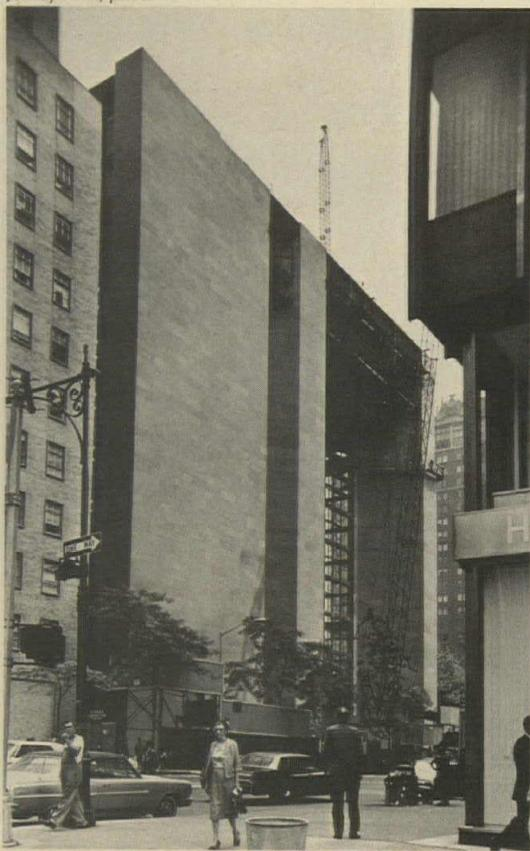
The Ford Foundation headquarters building, New York City, designed by Kevin Roche, John Dinkeloo and Associates, is nearing completion. The 10-story-high glass walls, which are hung from two upper floors, are now in place, enclosing a 100-foot-square skylit court. The 12-story granite-faced structure is in the shape of a "C" with right angle corners surrounding the garden court, which will also serve as an extension of an adjacent park. The general contractor is the Turner Construction Company.
