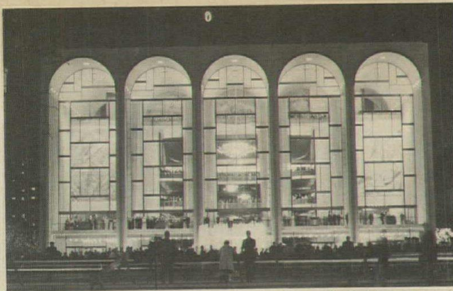
METROPOLITAN OPERA, Lincoln Center, New York City — Seven 8' x 60' stage lifts, two orchestra pit lifts, other equipment for handling sets and scenery.
