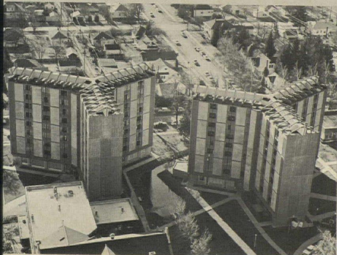
Precast floor panels are supported by hangers in tension rather than by conventional compression columns. The steel-strap hangers are stretched between outriggers at the top to grade beams at the bottom. The outriggers as well as the straps were fabricated from high-strength steel.
