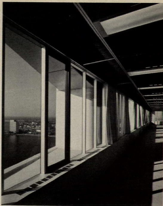
Mechanical equipment for air conditioning is located on the 9th and 20th floors. A special system of ceiling suspension beneath these floors consists of spring loaded vibration isolators which hold the framework for the acoustical ceiling and integrated lighting-cooling fixtures as shown above.
