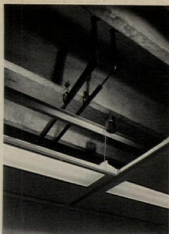
Mechanical equipment for air conditioning is located on the 9th and 20th floors. A special system of ceiling suspension beneath these floors consists of spring loaded vibration isolators which hold the framework for the acoustical ceiling and integrated lighting-cooling fixtures as shown above.
