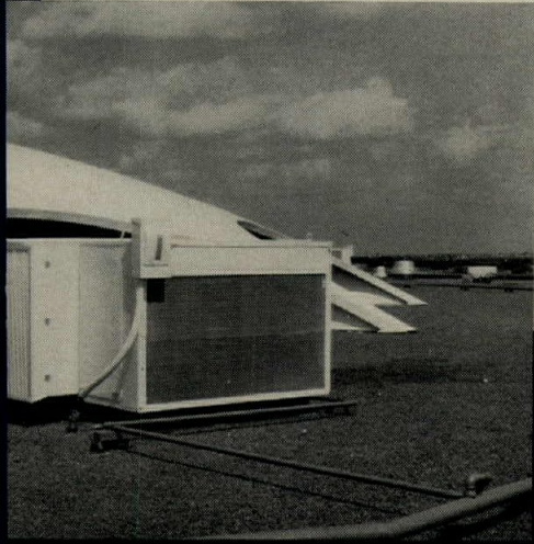
Design Concepts, John H. Glenn Junior High School, San Angelo, Texas: Plan view, above, shows how modern concepts of team teaching, flexible scheduling and individualized instruction find architectural accommodation. Roof mounted air conditioning equipment, with multizone distribution, permitted designers to eliminate "walls" of space and time. Thus, the building anticipates innovative teaching concepts of the future, as well as housing those of today. ARCHITECTS: Donald R. Goss Associates. ENGINEERS: Cowan, Love & Jackson, Inc. Four Lennox GCS3 single zone units serve large open areas in the center of the school. Capacity of each unit: 15 tons electric cooling; 200,000 Btuh gas heating.
