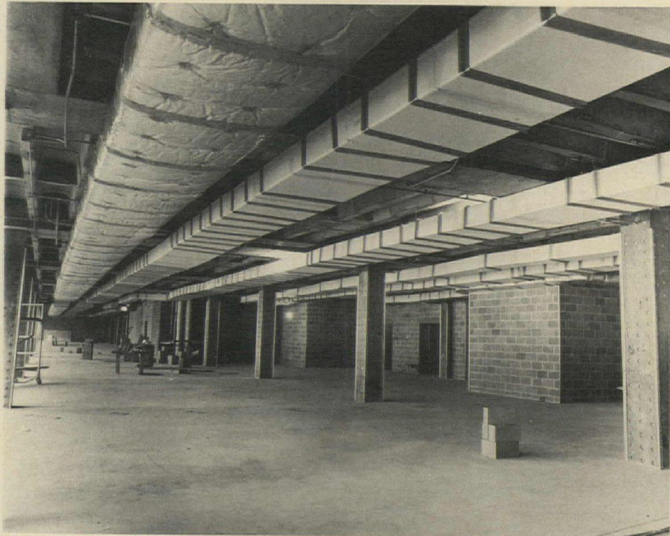
In the largest application to date, the Louisville Federal Building has fibrous glass ducts up to 37-in. wide, though for larger duct (at left in photo above) wrapped sheet metal was used. Typical fibrous glass duct sections, right, get T-shaped reinforcement and airtight tape sealing at joint.
