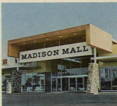
The mall of Rascoe-Tempo Stores, Fair Oaks, California, has an epoxy terrazzo floor based on Shell Epon resin. It has withstood over 3,000,000 shoppers since installation in December 1964.
