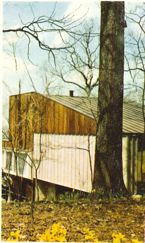
Hillside House, Baltimore, Maryland. Architect: J. William Ilmanen. Photo by Norman McGrath.
