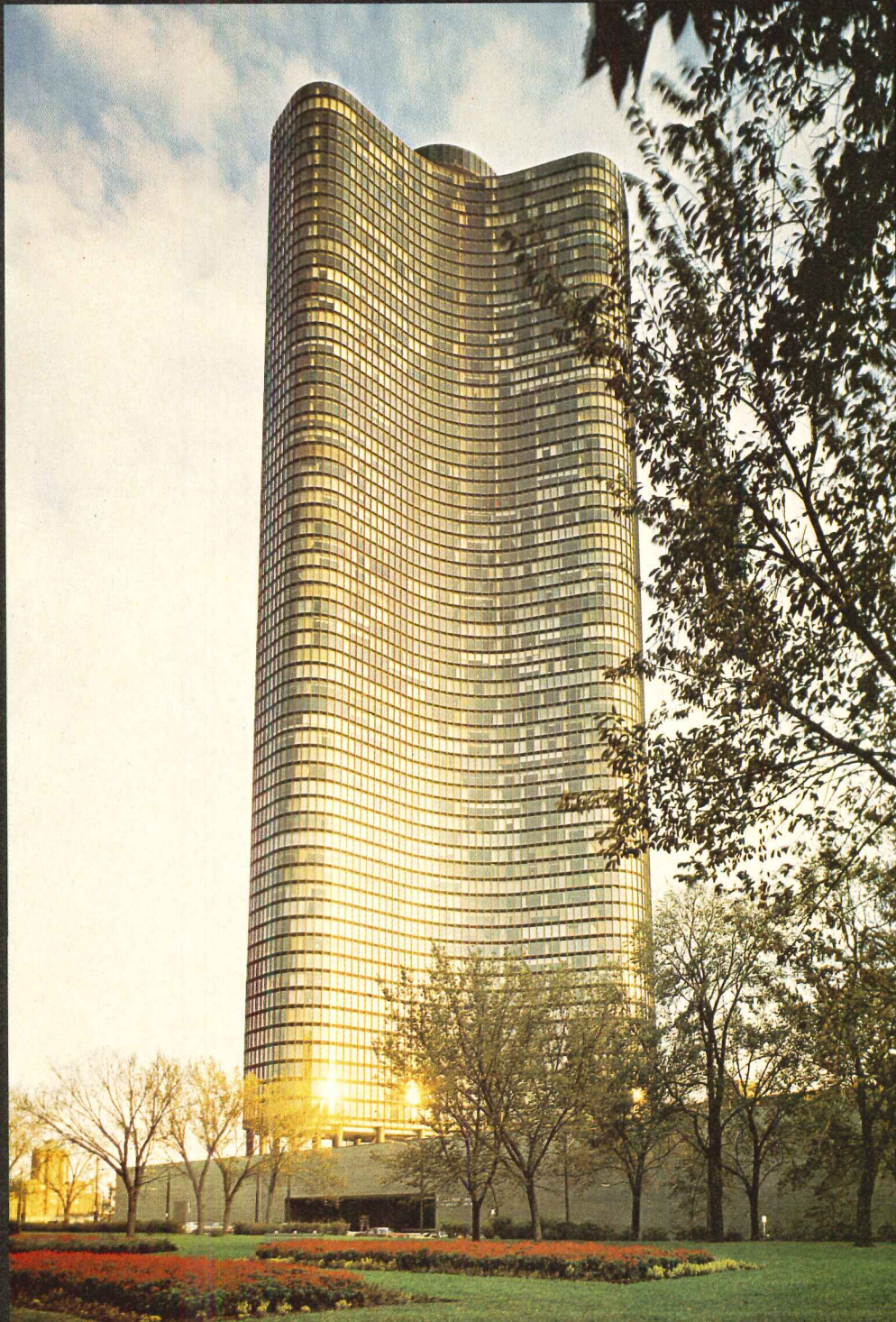
LAKE POINT TOWER, Chicago, Illinois/Architect: Schipporeit-Heinrich/ General Contractor: Crane Construction Co./Glazing Sub-Contractor: National-Hamilton, Div. of Bienenfeld Glass Corp. 1" Polarpane glazing manufactured by Polarpane Corporation
