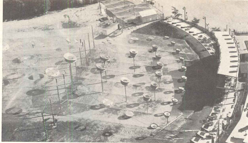
Stargets Golf Game, Hanover, Massachusetts Designer-Owner: Family Leisure, Inc., Engineering Consultant: Simpson, Gumpertz & Heger, Inc., Project Engineer: John F. Notemeyer, Steelwork: Chestnut Welding & Iron, Inc., General Contractor: Taverna Brothers
