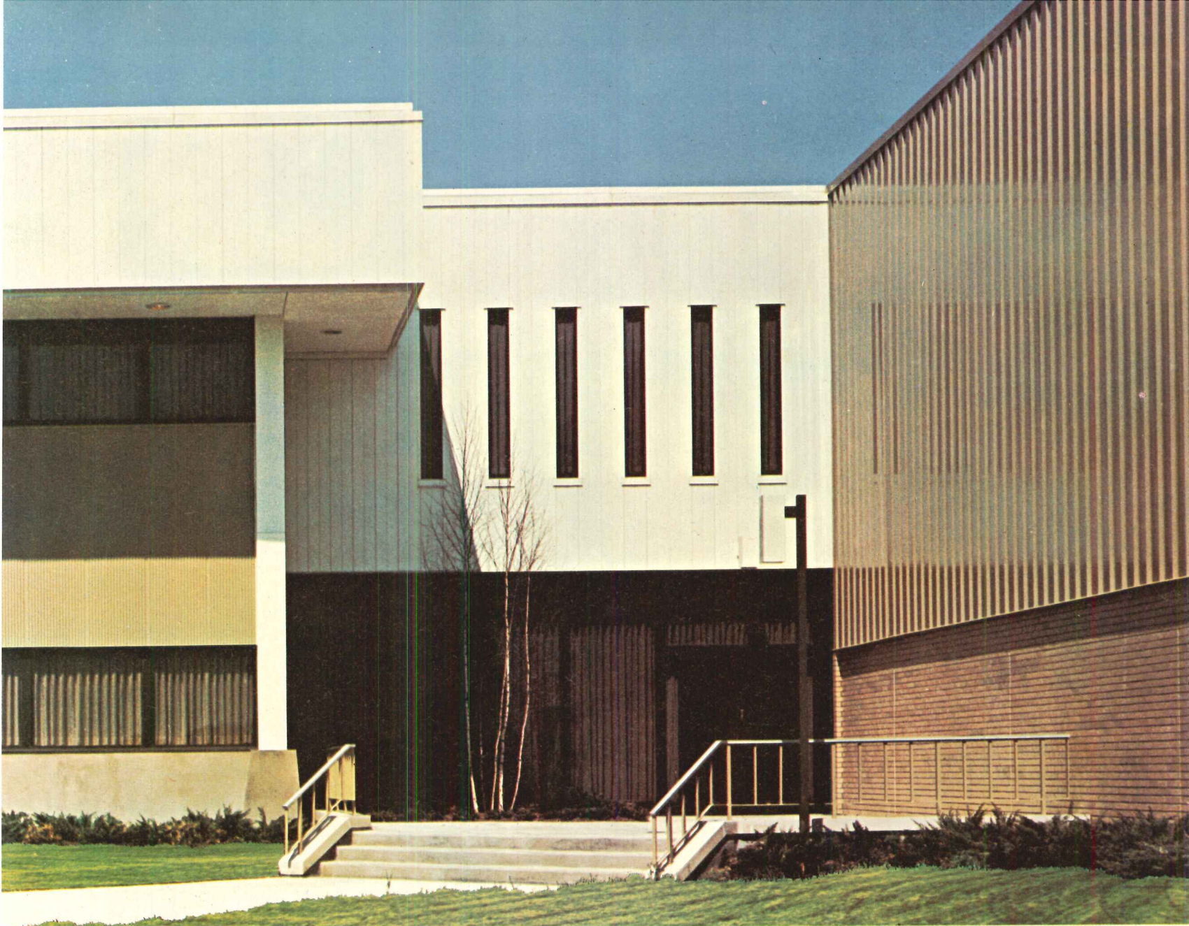
FMC Corporation, Packaging Machinery Division, Philadelphia Plant, Horsham, Pa.; Architects & Engineers: Alexander Ewing & Associates, Philadelphia, Pa.; General Contractor: Irwin & Leighton Inc., Philadelphia, Pa.
