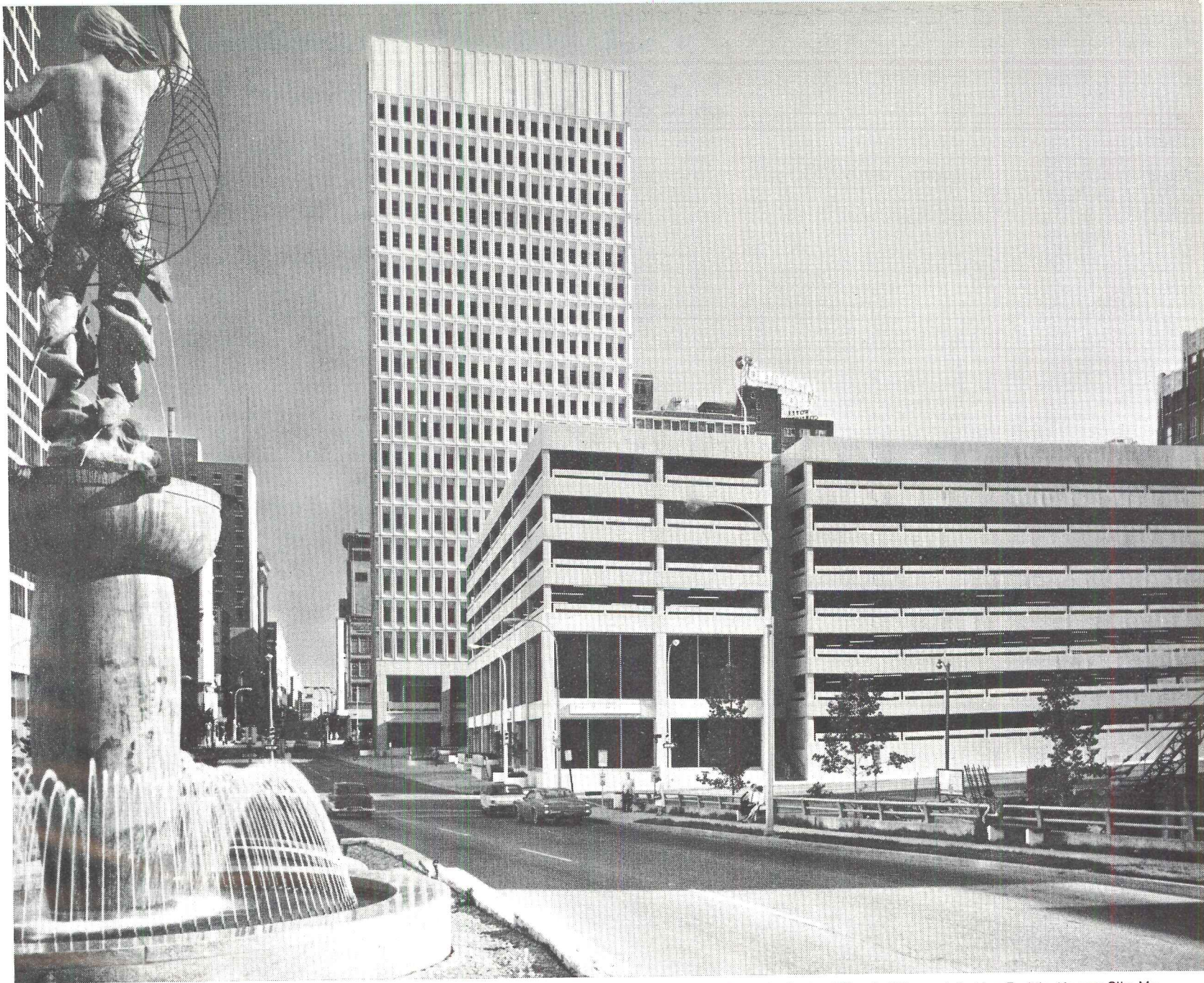
TenMain Center Office Building and Parking Facility, Kansas City, Mo. Monolithic reinforced concrete design/Robert P. Ingram, developer/Charles Luckman Associates, architects/Marshall & Brown, associate architects/Howard, Needles, Tammen & Bergendoff, engineers/Winn-Senter Construction Company, general contractor/506,354 sq ft of standard Ceco steelform services/2,900 tons of fabricated reinforcing bars by Ceco.
