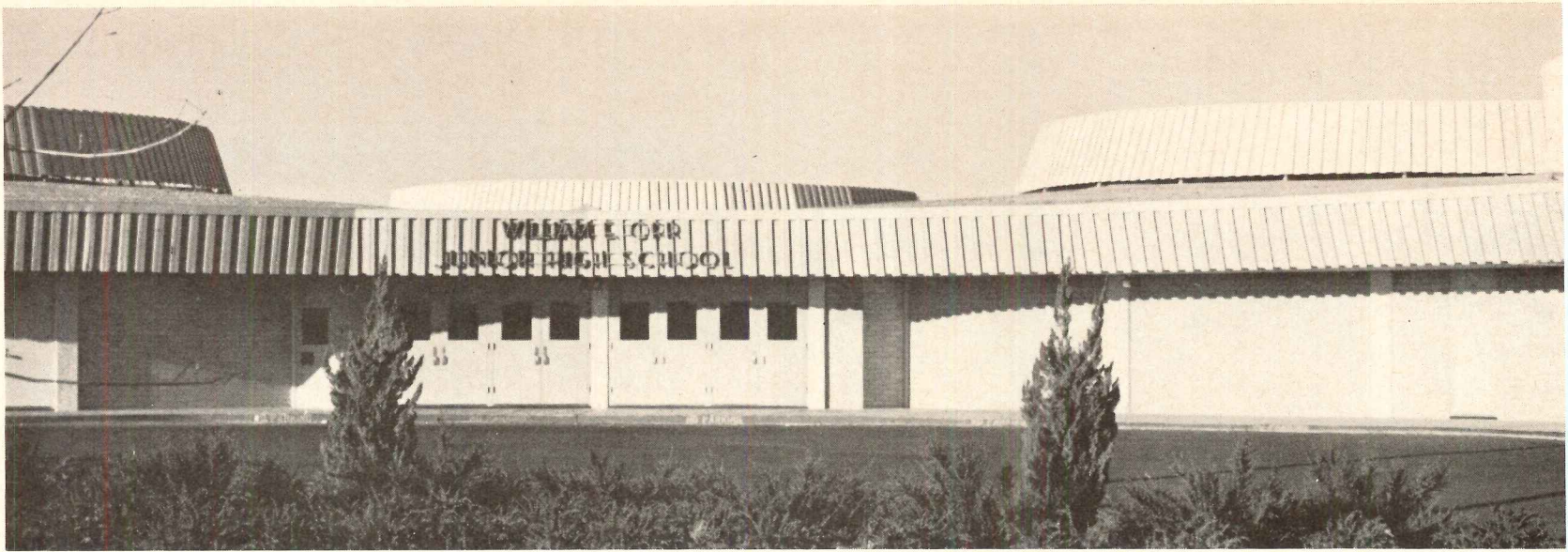
The low-profile Lennox DMS poses only a minimal screening problem. Example: The "pods" atop the William E. Orr Junior High School, Las Vegas, Nevada. Each conceals up to three DMS units. Architect: Zick and Sharp, in association with Shaver & Co. Engineer: Marvin Shafer.
