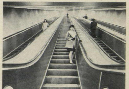
LONG ESCALATORS / Escalators 148 ft. long have been installed in a Tokyo subway station. They are sloped into the floor at a smaller angle for passenger comfort and ease in getting on and off. The elevators move at 90 ft/min and can carry 9000 passengers per hour. ■ Hitachi America Ltd., New York City.
