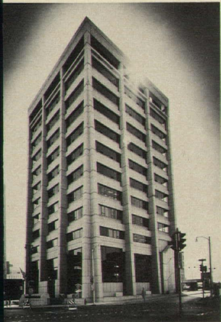
Continental Bank and Trust Co. , in Milwaukee, by Jordan Miller and George Waltz, Architects, A.I.A. and Associates, emphasizes its exposed concrete structure. The tapered wind-bracing exterior columns compensate for the removal of the service core to one side, allowing for maximum open space on the main banking floor.
