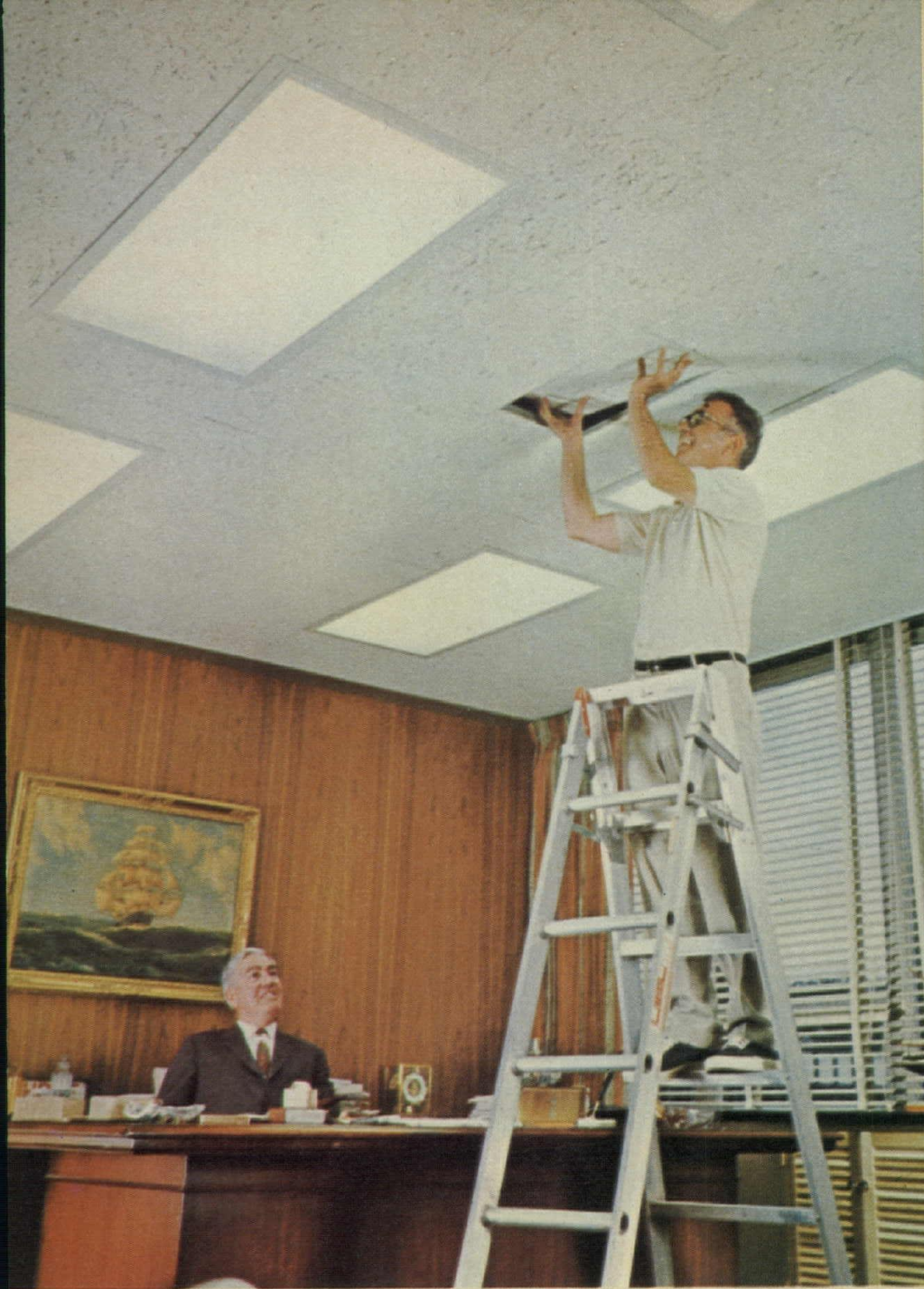
In corporate headquarters offices of Heublein, Inc., in Hartford, Conn., tiles fit snugly in the Accesso Concealed Suspension System to form a smooth, almost seamless ceiling.
