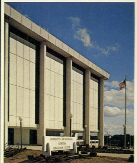
This crisp, modern facade belongs to the Education Center for the Charlotte-Mecklenburg Schools in Charlotte, North Carolina.
