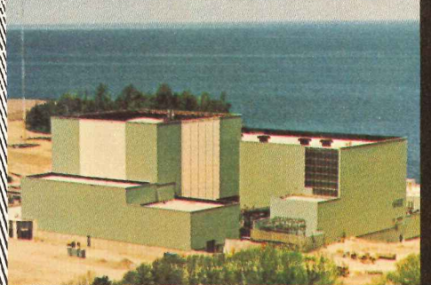
1. Ginna Nuclear Station, Rochester Gas & Electric Corp.
