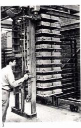
1) The pug mill where the clay is mixed and kneaded. 2) Hand-throwing into molds. 3) All handling is by conveyor belt or pallets. 4) The bricks ready for firing. 5) Finished product.
