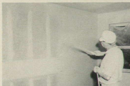
Hide-A-Spray Latex paint completely covered taped and spackled joints in dry-wall in one pass of the airless gun.
