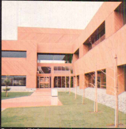
Redwood T&G lumber applied diagonally on office building complex
