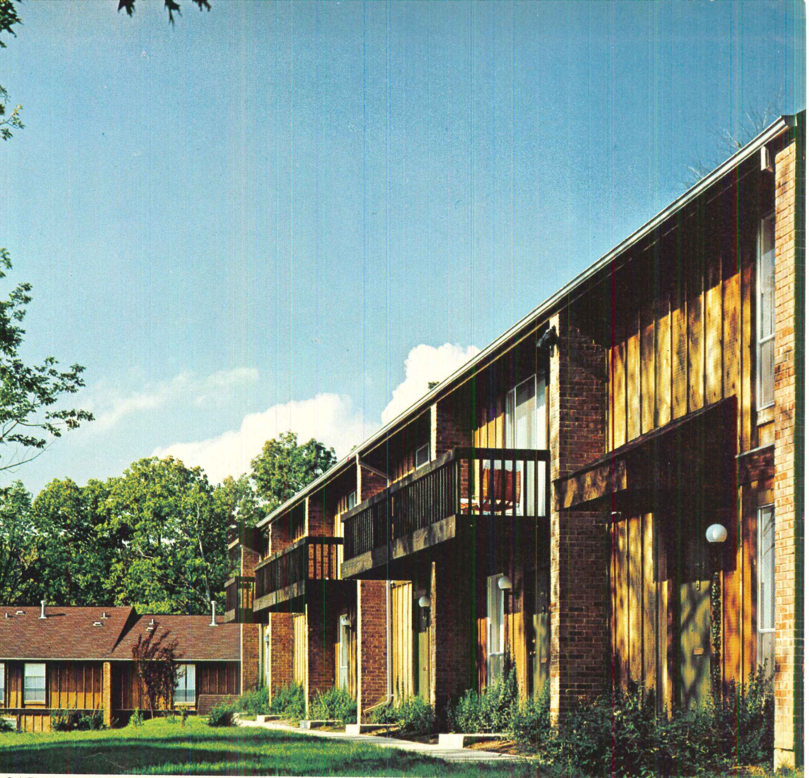
For Oak Townhouse and Apartment complex, St. Louis, Missouri, features use of Non-Com® Exterior for board and batten cedar siding. Owner: Lincoln Property Company, St. Louis. Architects: Dale E. Selzer, AIA, Dallas; Hastings and Chivetta, AIA, St. Louis.
