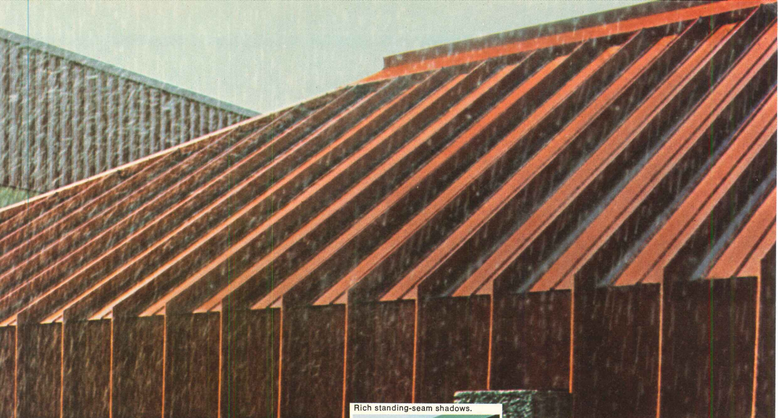
Continuous ridge-to-eaves lengths without endlaps.
