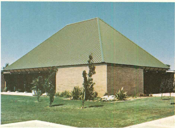
An attractive, tight hip roof.
