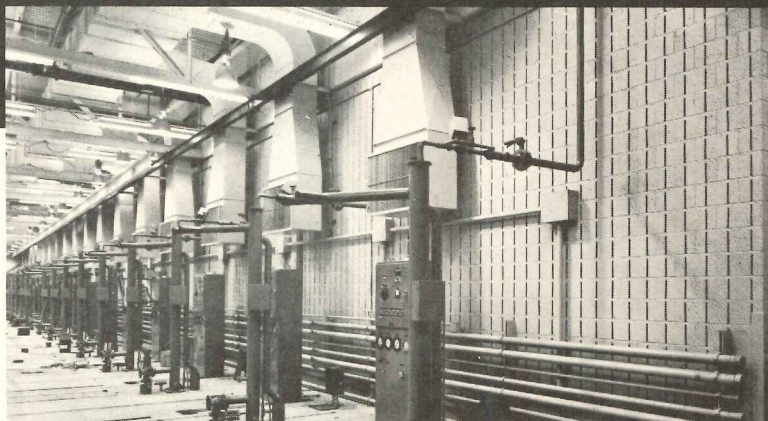
85,000 SOUNDBLOX Units Quiet This General Motors Corporation, Detroit Diesel Engine Division, Test Facility. Architects: Argonaut Realty Division, G.M.C.
