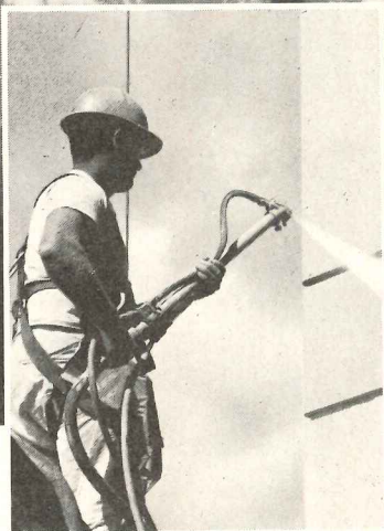
MODULAR HOUSING: Today's trend in modern housing—easily erected modules grouped according to specifications. These attractive units were permanently decorator-finished with cement-base THOROSEAL PLASTER MIX sprayed on with the versatile, dependable Thorogun. It sprays up to a 27" swath for fast, efficient applications. (Photo by R. M. Liselen)
