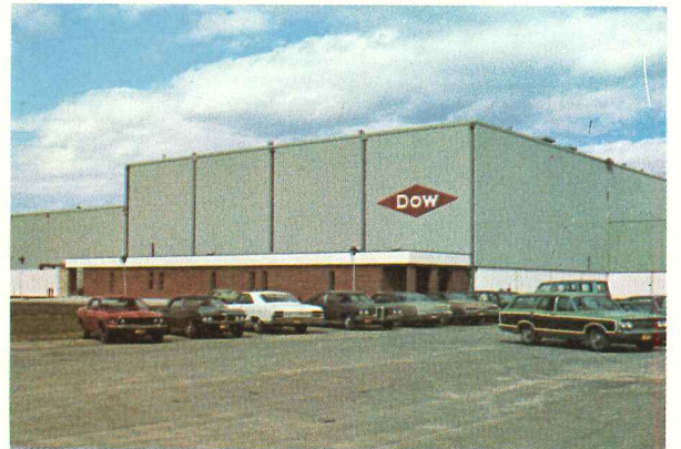
The Dow Chemical Company, Newark Ohio Industrial Park, Newark, Ohio. Architect: Curtis N. Lindberg, Columbus, Ohio. C-Panel System, Shadowwall Exterior Profile.
