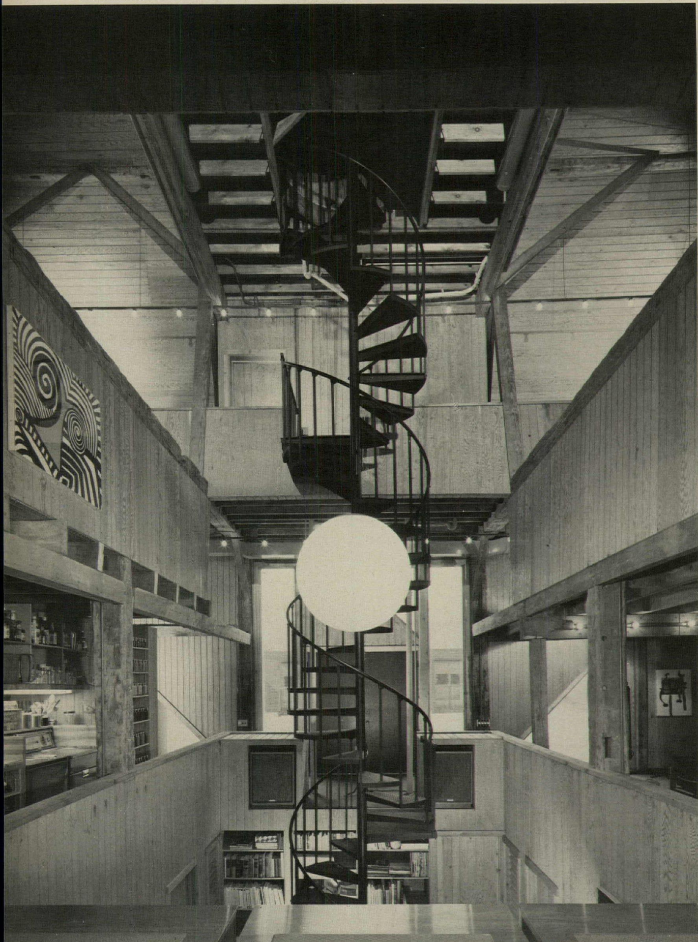
The freestanding circular metal stair connects all levels serving as the dominant sculptural element
