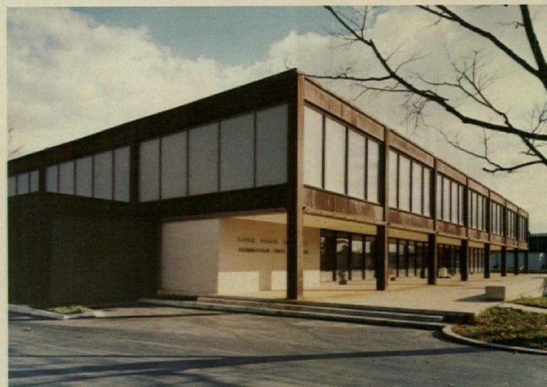
FOURTH DISTRICT HEADQUARTERS, METROPOLITAN POLICE DEPARTMENT, Washington, D.C. Jurors' Comment: "The jury regards this dignified design for a government agency as having considerable importance. It represents a trend toward simplicity and direction that should be recognized and encouraged."
