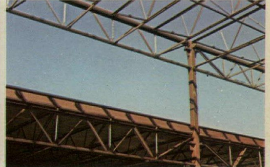
The light weight and simplicity of Vulcraft's steel joists and joist girders make erection fast and easy.
