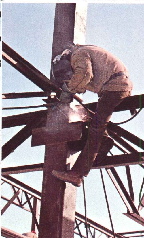
Vulcraft steel joists and joist girders allowed for simple and fast column connections.
