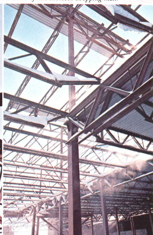
Joist girder design flexibility provided for a wide range of load support, from normal roof loads to heavy mechanical equipment loads.
