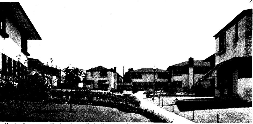
Housing Group, Jersey City, New Jersey; Charles Shilowitz, architect; March 1937 (George H. Van Anda)
