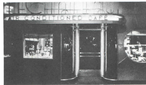
1 Restaurant entrance, Fargo, North Dakota; Paul W. Jones, architect; January 1939.
