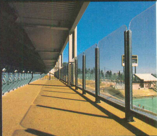
Spectator glazing protects without obstructing view of game at University of Colorado Stadium, Boulder, Colorado. Architect: Herb Ross.
