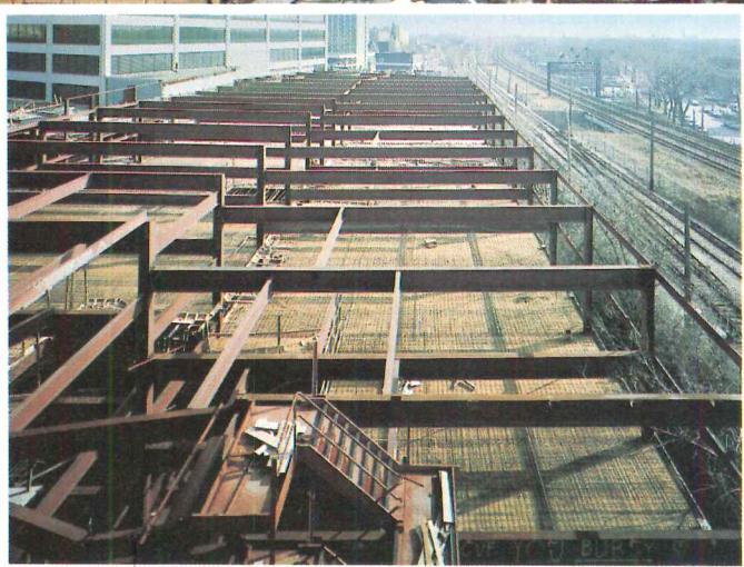
Parking deck structure.
