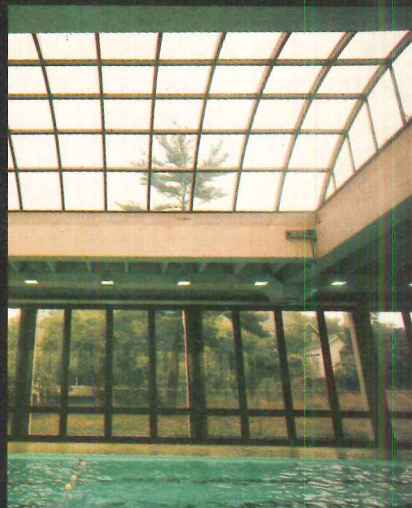
This skylight is representative of the type of skylights now being fabricated with "Lucite" cast acrylic sheet.
