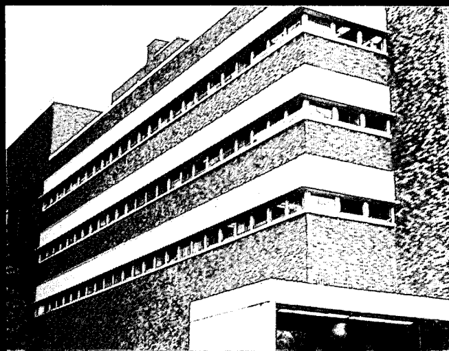
Sun Shades, University of Washington. Architect: Shavey & Schmidt. Manufacturer: Olympian Stone Co., Redmond, Washington.
