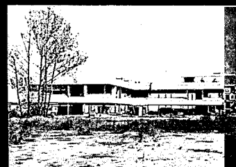
Aggregate faced panels in a variety of sizes from 3' x 3' to 12' x 9' for a MetroCenter office building, Nashville, Tenn. Architect: Hart, Krivatsy & Stube, New York, N.Y. Manufacturer: Cem-Fil Corporation, Nashville, Tennessee.
