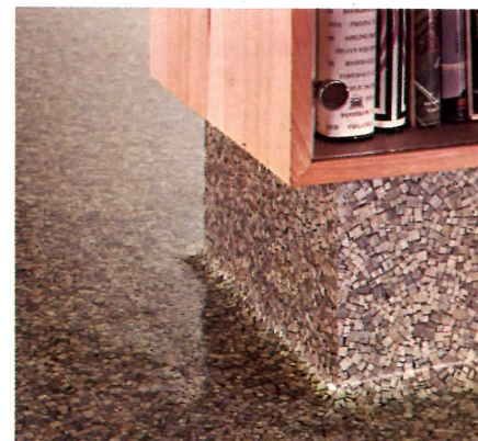
Brigantine can be covered where the floor meets the wall to help eliminate places where dirt can hide.
