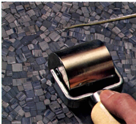
Seams are chemically welded to provide a continuous surface that resists penetration of dirt and moisture.
