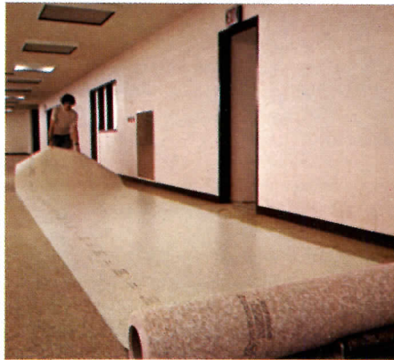
Rolls 6' wide and up to 90' long keep seams to a minimum, provide an almost monolithic look.
