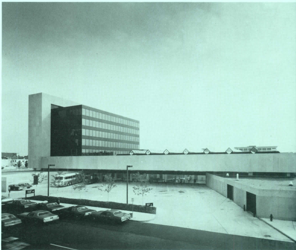
The Metropolitan Transportation Center in Buffalo, New York, consists of a low-slung, skylit section, housing a concourse for the bus terminal, and a mid-rise office building, housing the administrative functions of the area's transportation authority. Cannon Design, Inc., the architect, has laid out and detailed the place with care, clarity, and a determination to allow the movement of people and the movement of light to assume the role of art. Graphics, though eye-catching, are as constrained as they are expressive in this limestone-and-glass pavilion.
