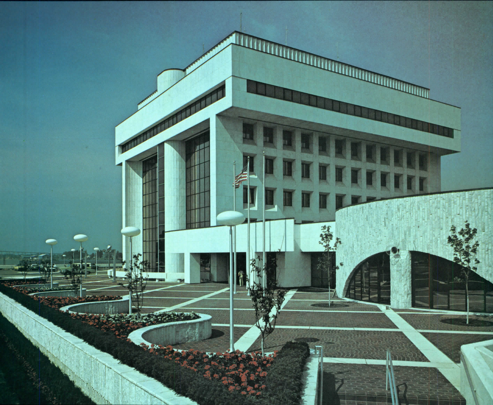
Port Huron Municipal Office Center Building, Port Huron, Michigan | Arch: Richard C. Cogley | All white material in photo is Cherokee marble, supplied by Genesee Cut Stone & Marble Co., Flint, Michigan
