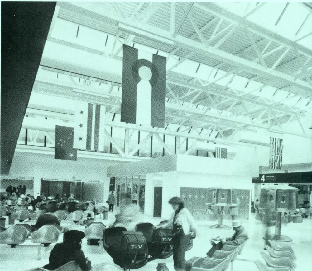
Spanning the terminal concourse of Buffalo's Metropolitan Transportation Center is a series of exposed steel trusses, 140 feet long, and these are cantilevered outside for covered access to the buses. A series of skylights, running above the trusses, admit lots of natural light, dappling the interior with plentiful, changing moods. A roof garden, on the second level, overlooks this busy room, creating a spatial hinge between the horizontal element of the concourse and the vertical element of the adjacent office building. Views south take in the city's rich architectural heritage.
