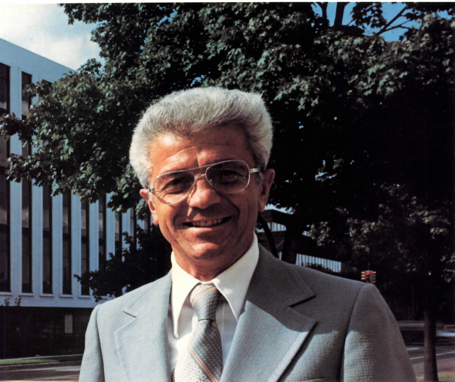
1050 Franklin Avenue Building's impressive front entrance is accessible from the adjoining parking lot. The 6-level structure contains 69,600 sq ft of rentable space. Bethlehem's preliminary frame analysis indicated that high-strength steel and composite construction would best satisfy the owner's requirements.
