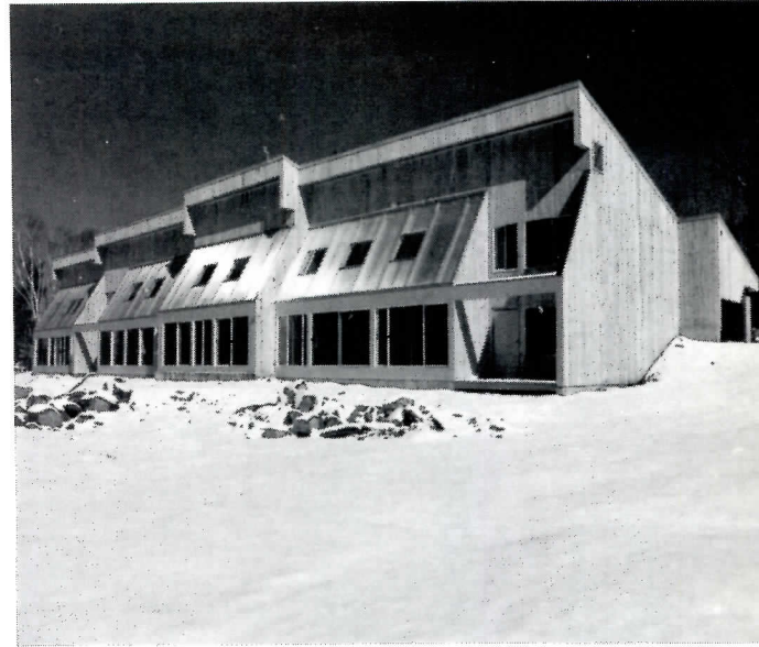
Sloped glazing for passive solar in this housing at White Mountain School in New Hampshire has clear panels for a view of the sky in the midst of a large area of panels comprising acrylic double-skinned sheet made by Cy/Ro Industries (winter U value is 0.58). Architects: Banwell, White and Arnold.
