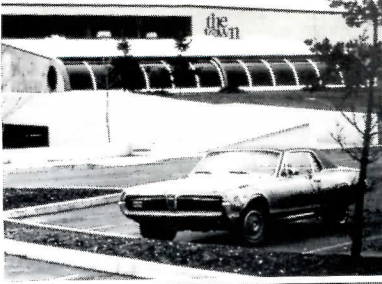
The translucent "skyroof" over this fast-food restaurant in Portland, Oregon is the first application of a translucent roof covering that has a Class "A" U.L. listing (for severe fire exposures). It comprises fiberglass-reinforced plastic skins bonded to an aluminum grid by Kalwall Corporation. Architects: Boutwell, Gordon, Beard & Grimes.
