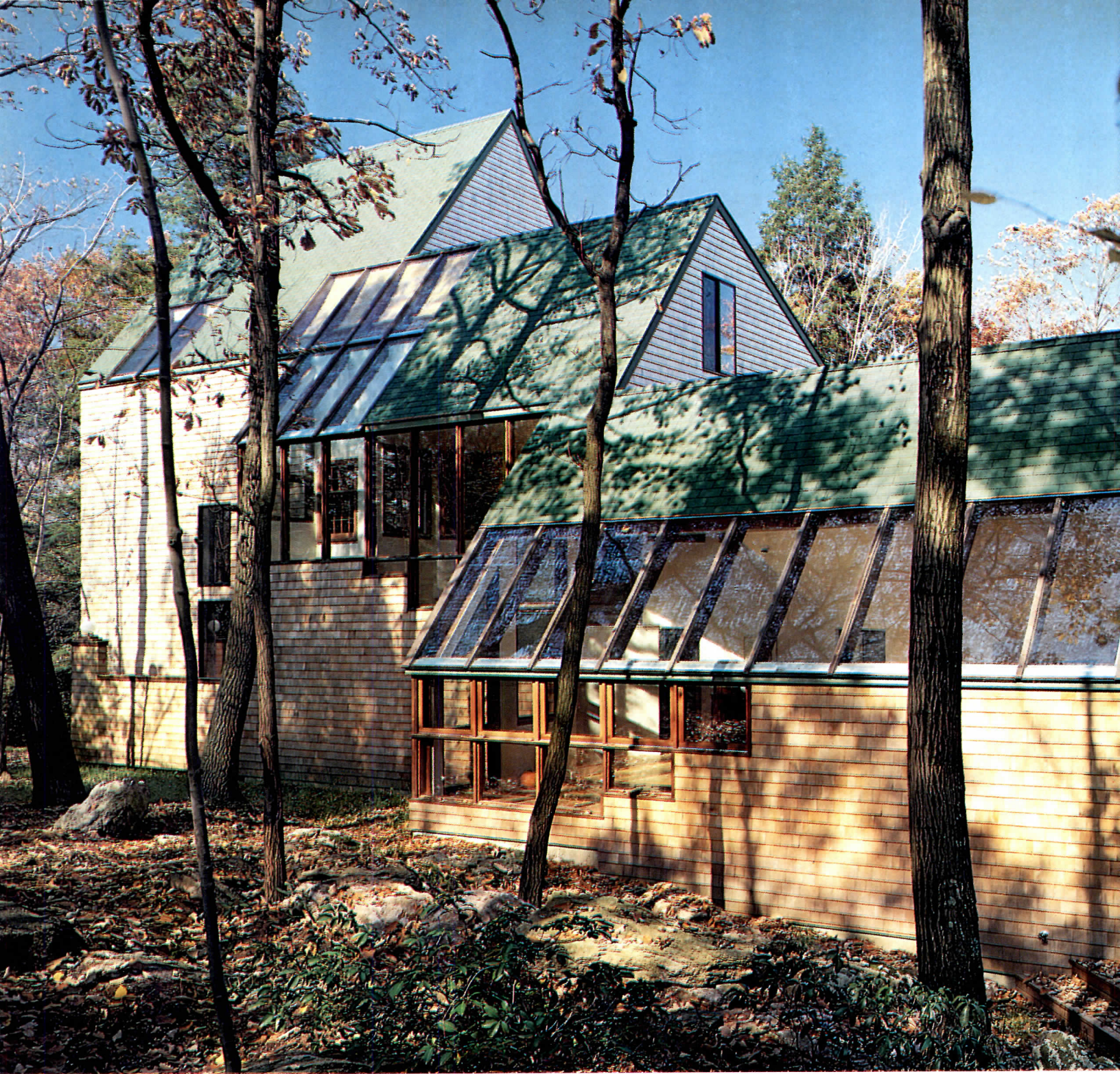
Percarpio Residence Southern Connecticut Moore Grover Harper, Architects
