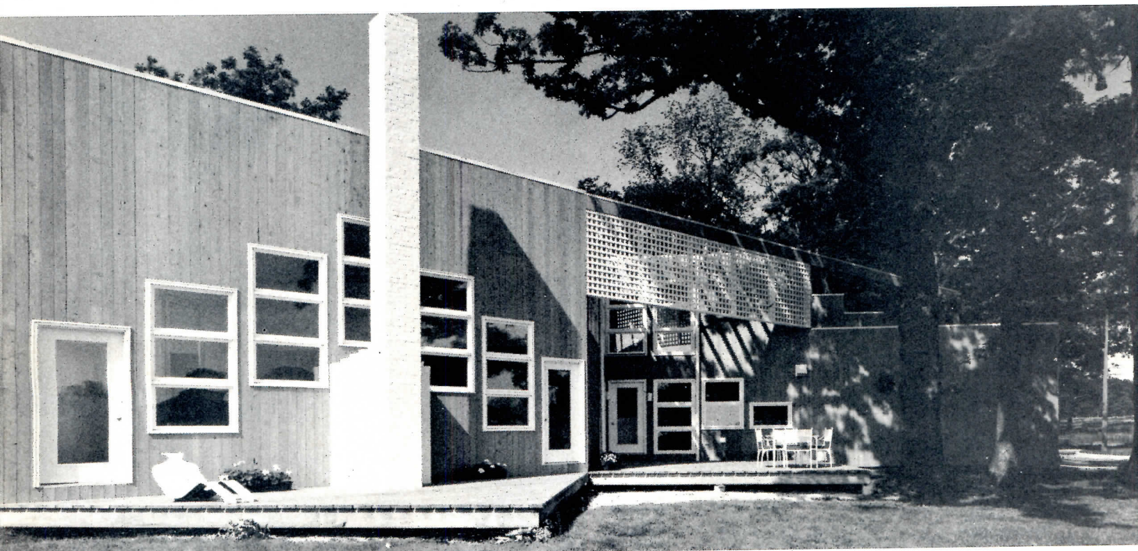
Marion house Lisle, Illinois Stanley Tigerman, Architect
