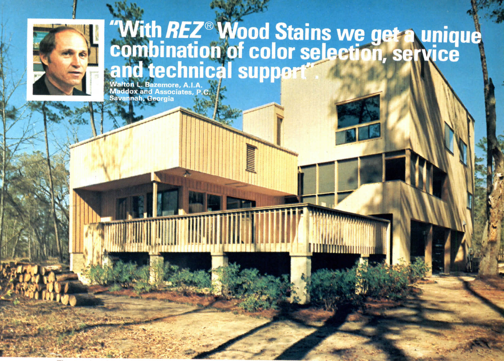
The exterior of this striking home designed by Walt Bazemore is made entirely of cypress and stained with REZ Oil Type Semi-Transparent Wood Stain. A variety of Pittsburgh® Paints were also used throughout the interior.
