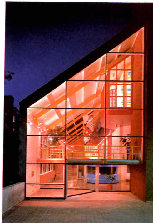
The circulation corridor that joins the new Ainsworth Gym to the older Scott Gym to its east dominates these views of the north facade. Rising beside the trapezoidal opening is the north stair tower.
