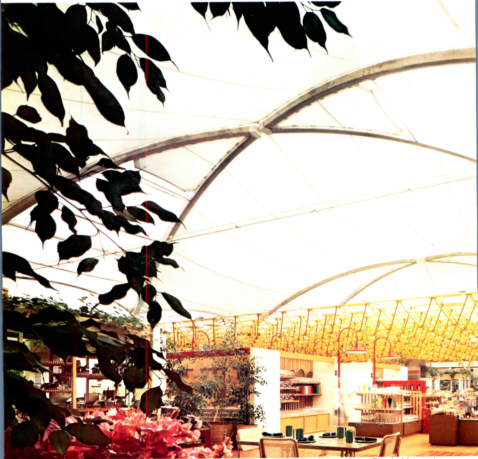
Bullock's, San Jose, California—the world's first department store under a permanent Owens-Corning Fiberglas fabric structure. Environmental Planning and Research, Inc., architects and planners. Geiger-Berger Associates, structural engineers.
