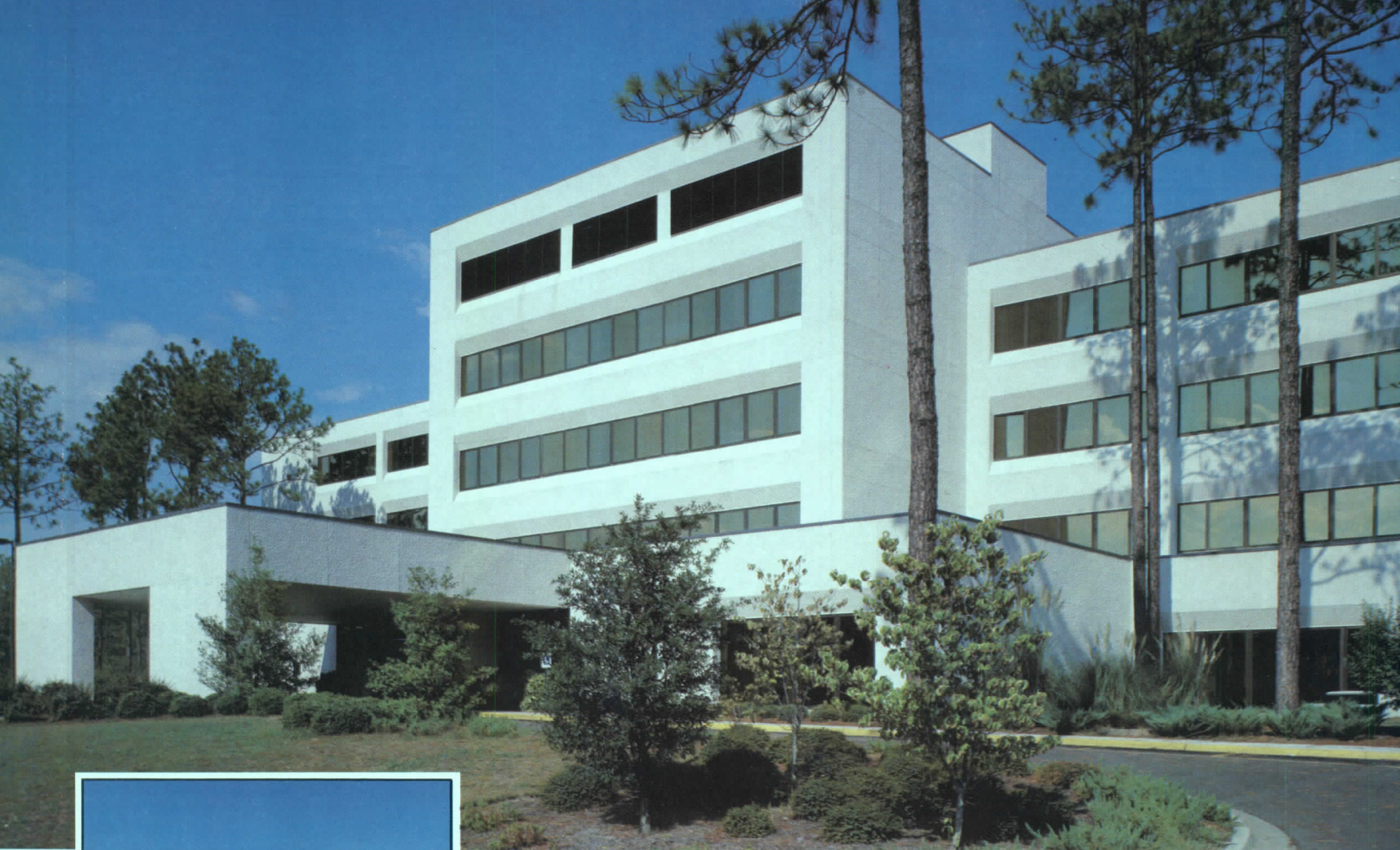
Aiken Community Hospital Aiken, SC - Architect — Gresham & Smith
