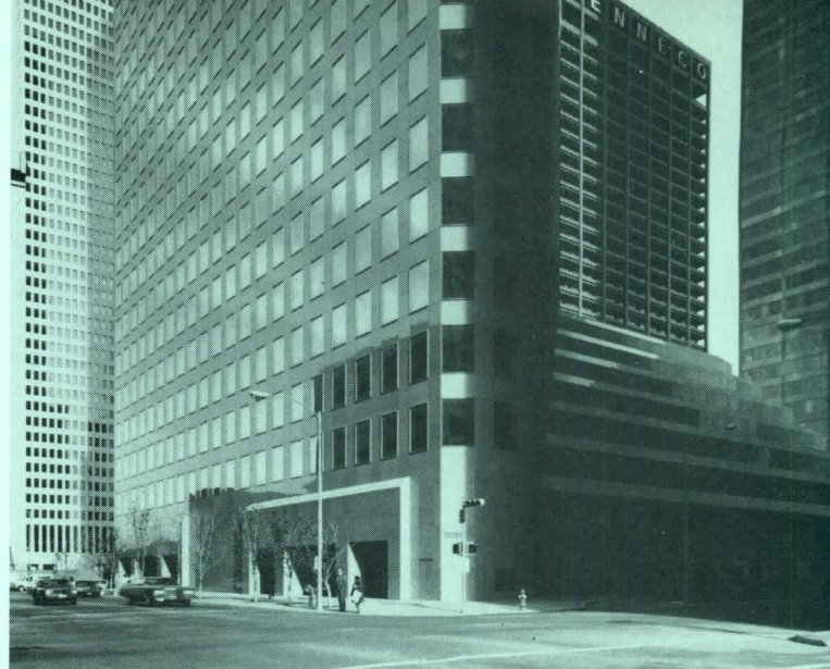
The L-shaped First International Plaza has a 55-story-high tower with a low-rise attachment for a banking hall, seen prominently from the street (below). One elevation (right) is intricately beveled front to an open plaza while reflecting light differently than any other building in town.
