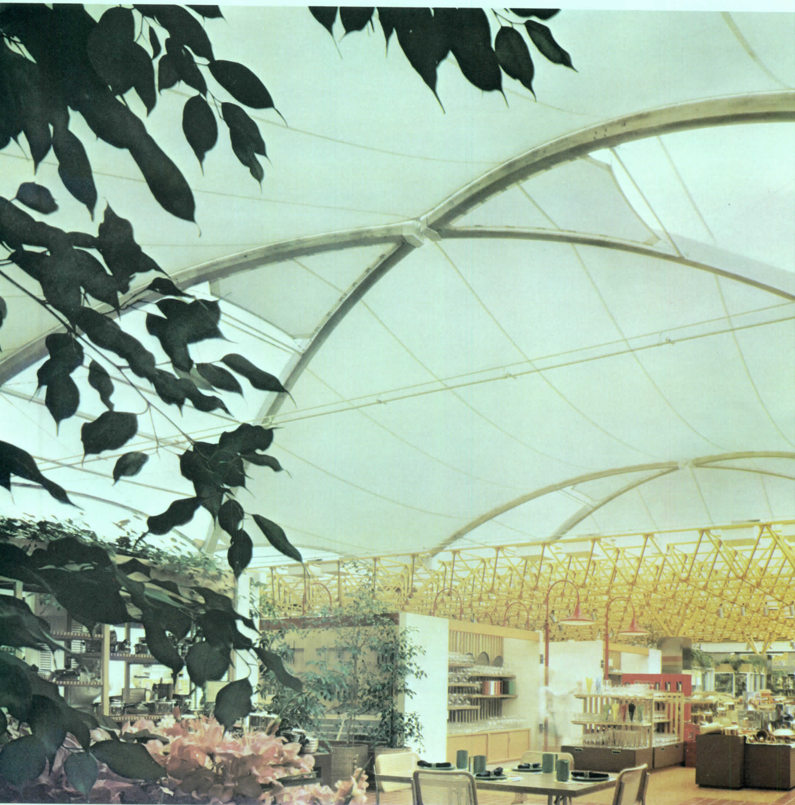
Bullock's, San Jose, California—the world's first department store under a permanent Owens-Corning Fiberglas fabric structure. Environmental Planning and Research, Inc., architects and planners. Geiger-Berger Associates, structural engineers.
