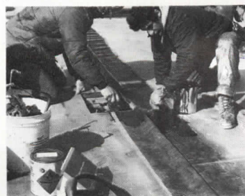
2 Stress forces, as shown in the drawing above, challenge roofers to make their field seams with care. Shear stresses, caused by expansion or contraction of a building or the movement of insulation materials or other substrates such as decks, can deform seams, subjecting them to peel forces as well—to which they have less resistance. The
