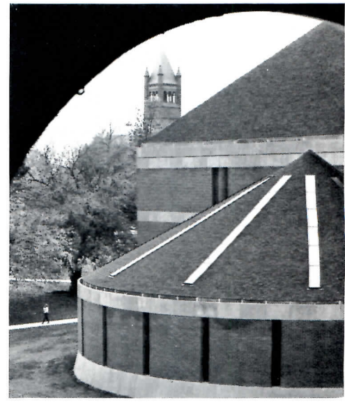
Finger skylights on apsidal roof, Library and Learning Center, Gettysburg College, Pennsylvania
