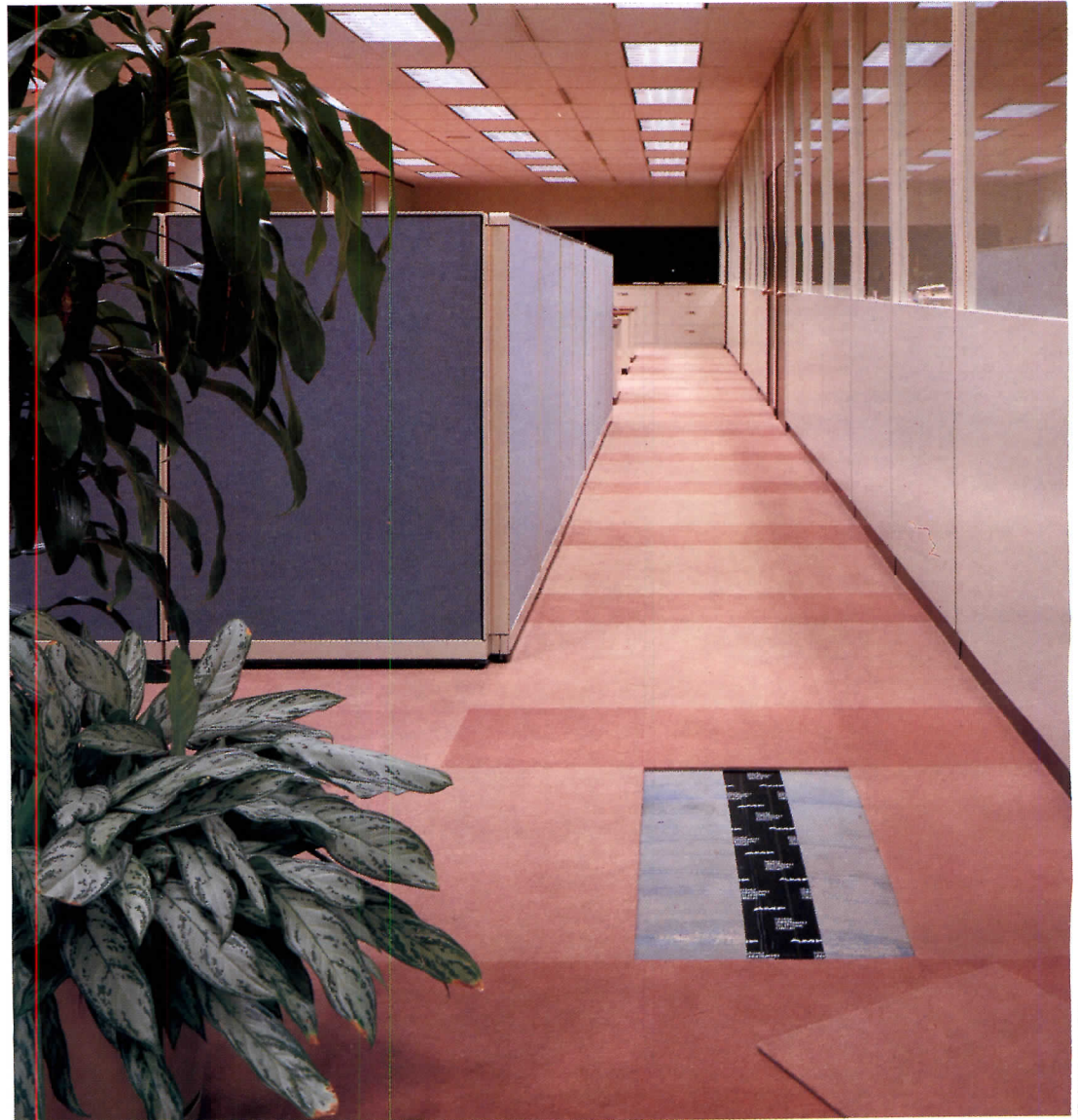
Photo 24: model P5300 Series fusion-bonded carpet tiles over flat telephone cable, installed at AMP Inc., Schaumburg, Illinois, Interface Flooring Systems; figure 25: construction of fusion-bonded carpet tile, Interface; photo 26: fusion-bonded carpet tiles, Milliken & Company.
