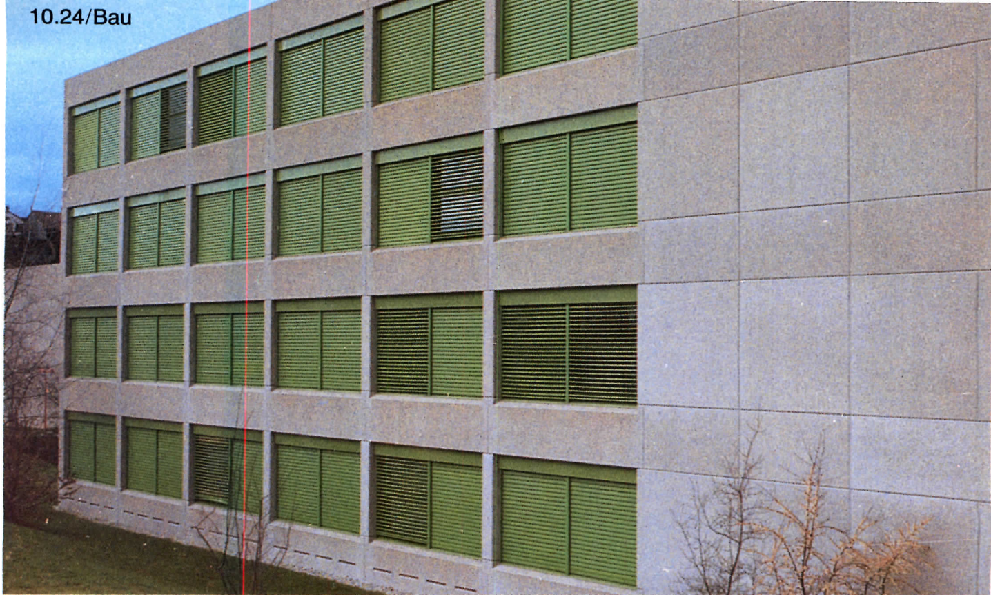
Above, weekend overtime workers in various offices use local override controls to open own blinds to enjoy natural daylighting.
