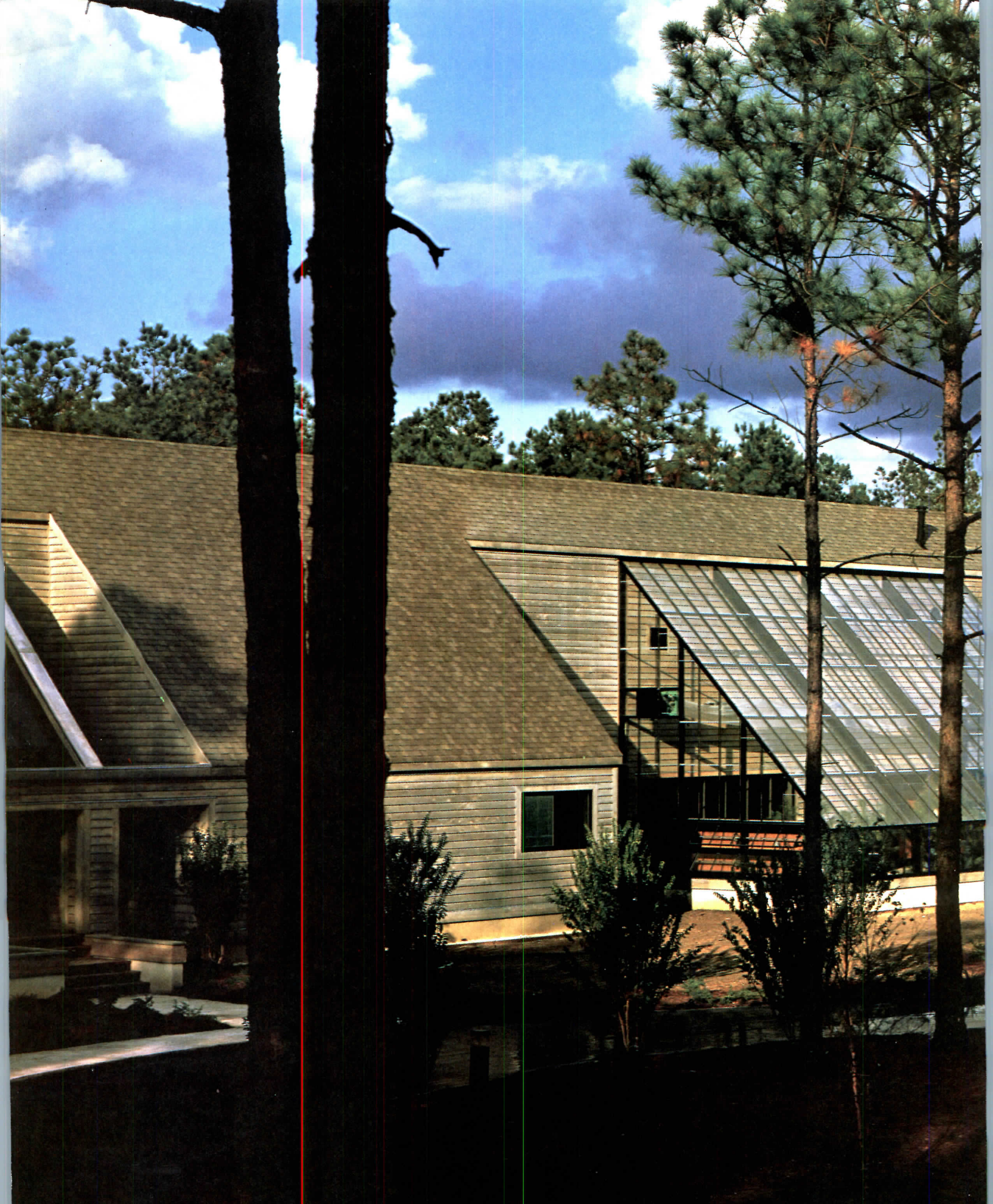
Westvaco Forest Science Laboratory Summerville, South Carolina Lucas Stubbs Pascullis Powell & Penney Ltd., Architects
