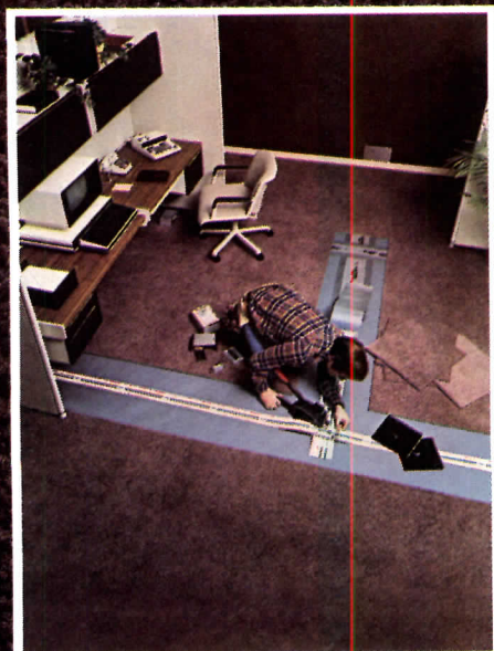
Flexway Undercarpet Systems for power, telephone and data transmission.
